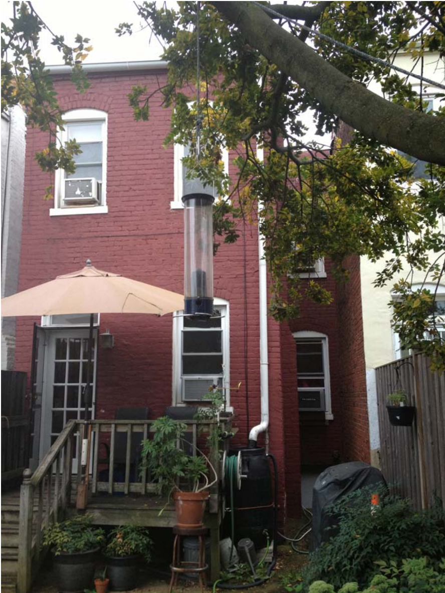
Existing Non-conforming Open Court
