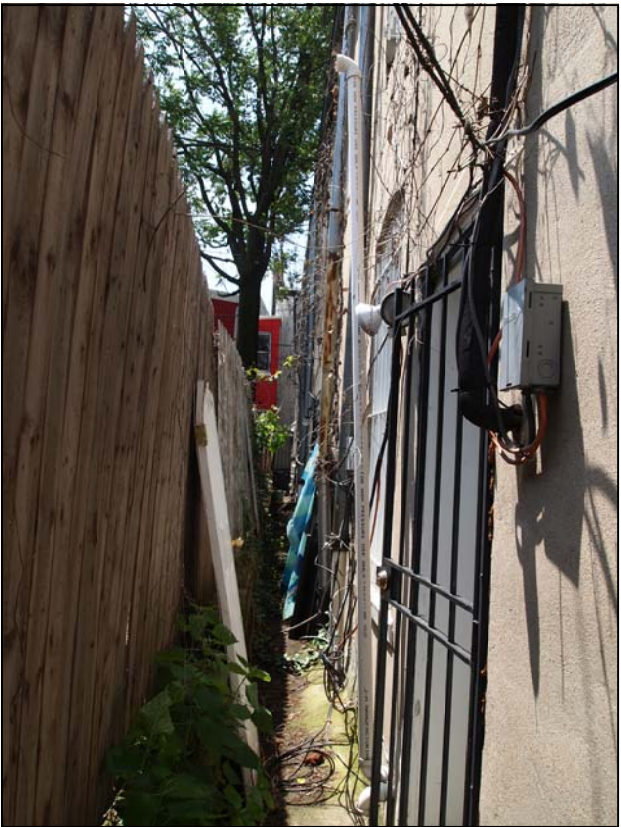
4 AREA B/W REAR WALL AND PROPERTY LINE
