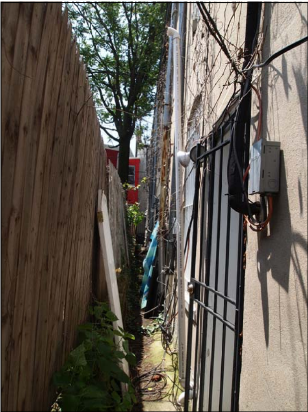
4 AREA B/W REAR WALL AND PROPERTY LINE
