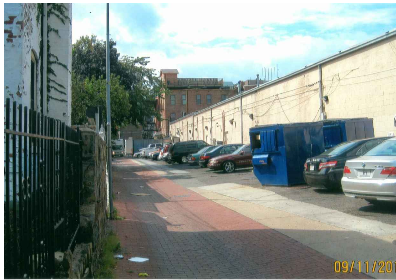
VIEW 6 ACROSS STREET REAR ELEVATION
