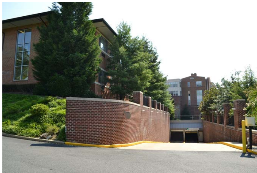
4. ENTRY TO EXISTING UNDERGROUND PARKING
