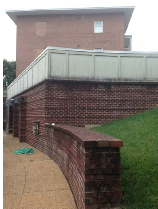
2. LOOKING SOUTH AT McCRACKEN
