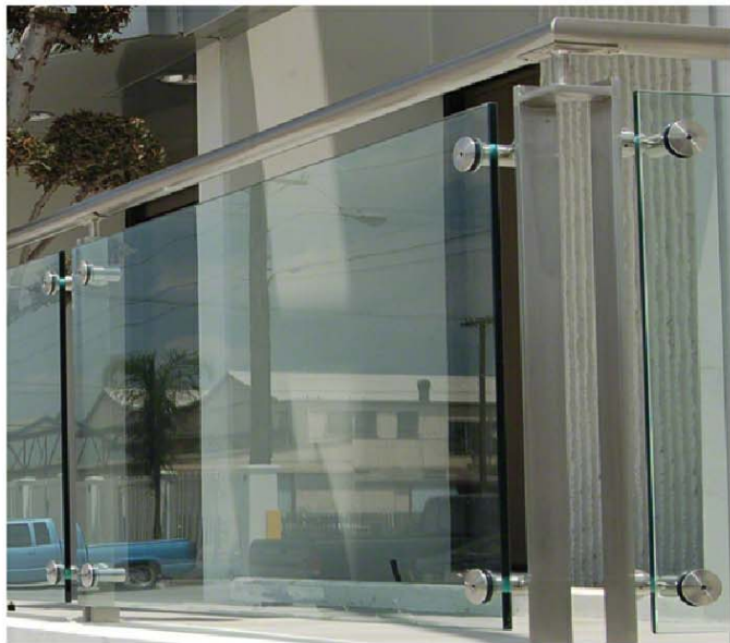
GLASS RAILINGS WITH STAINLESS STEEL TRIM
