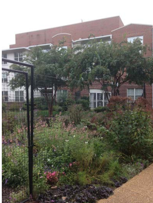
1. LOOKING SOUTH AT EXISTING IL BUILDING 6
