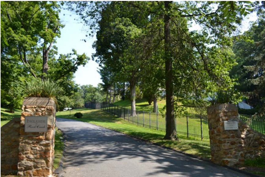
1. ENTRY DRIVE LOOKING FROM BROAD BRANCH
