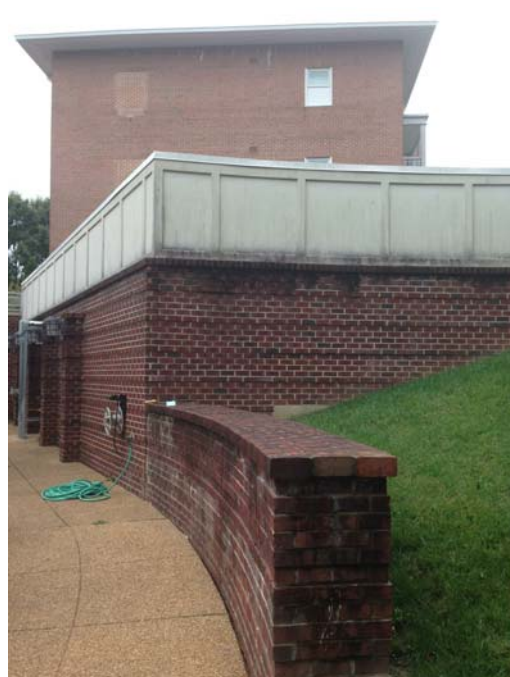
2. LOOKING SOUTH AT McCRACKEN
