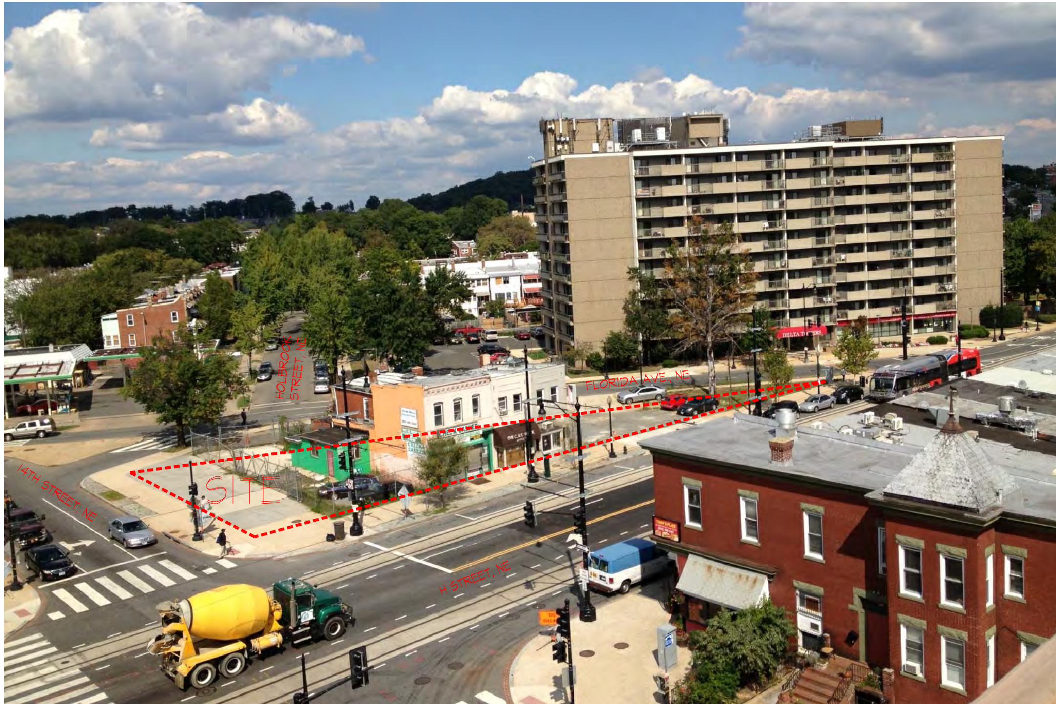
AERIAL VIEW FROM THE SOUTH-WEST
