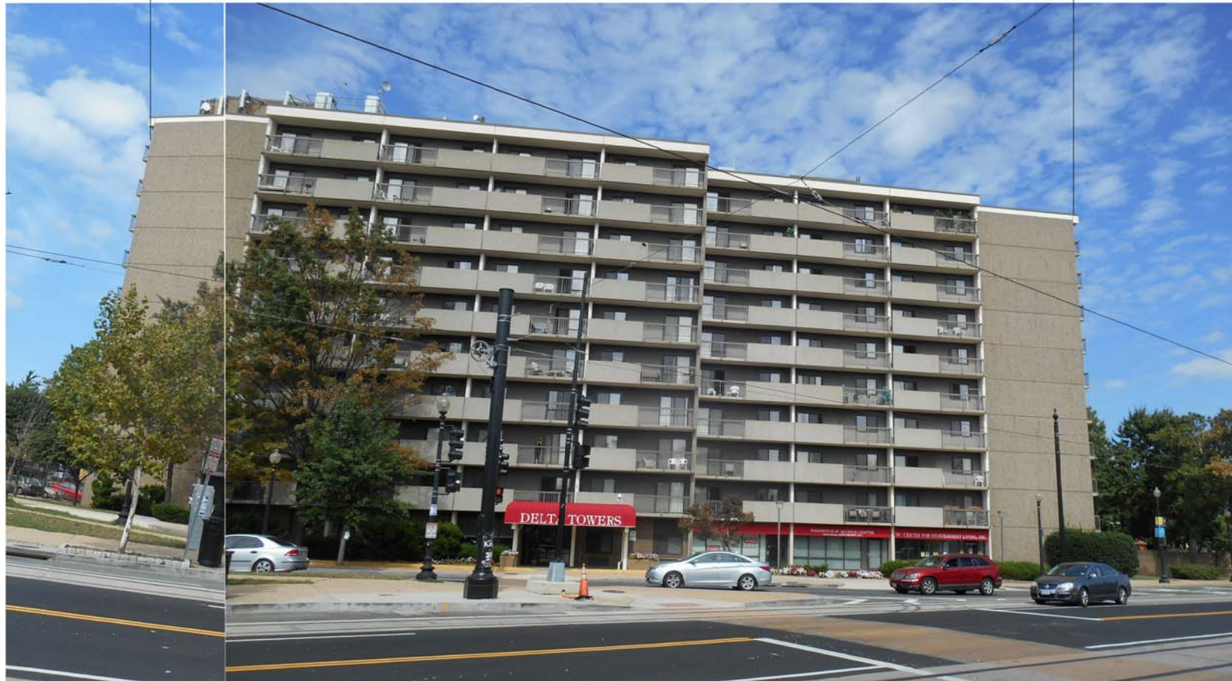
01. VIEW FROM ALONG FLORIDA AVE NE, LOOKING NORTH
