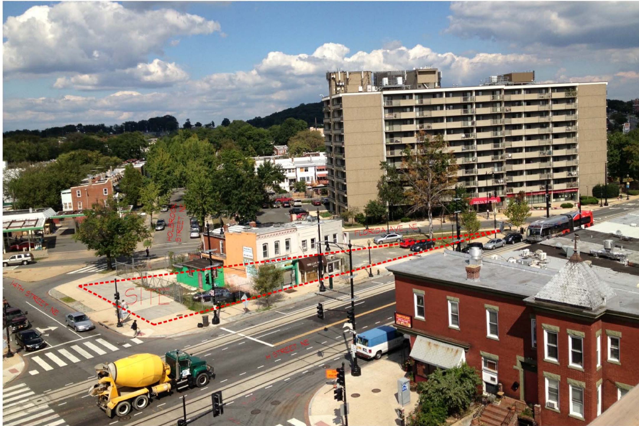
AERIAL VIEW FROM THE SOUTH-WEST
