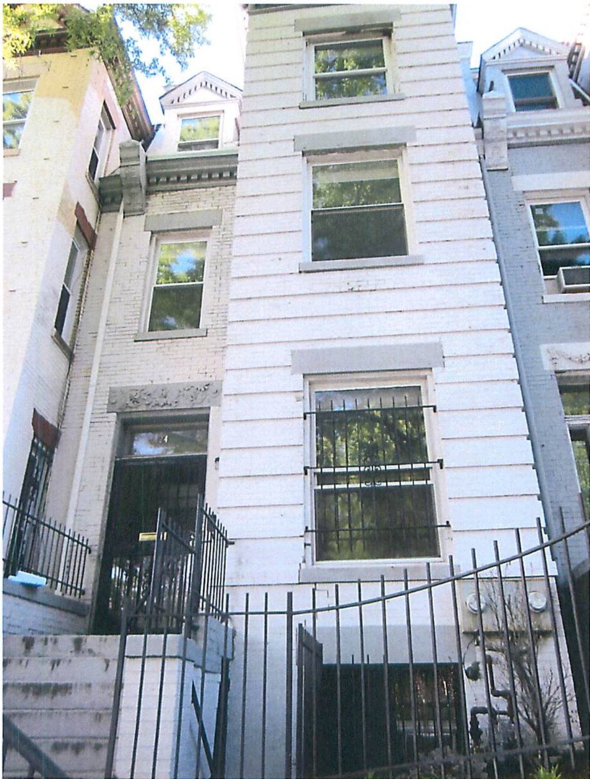
24 Rhode Island Ave NE Front Elevation to Remain
