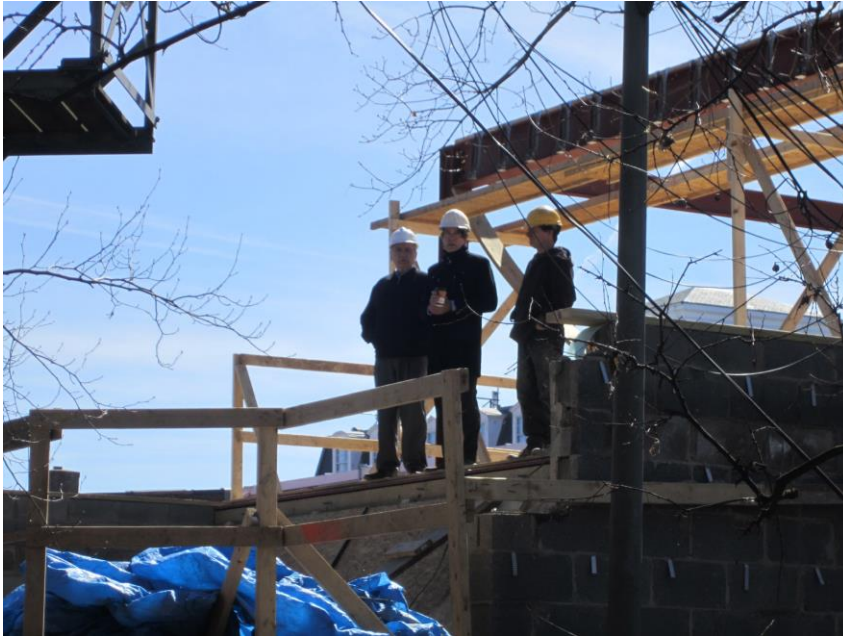
Mr. Bell looking into Junker kitchen
