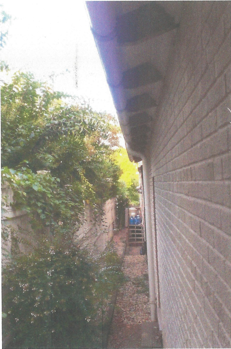
North Side of the Structure, Adjacent to 2808 34 th Place
