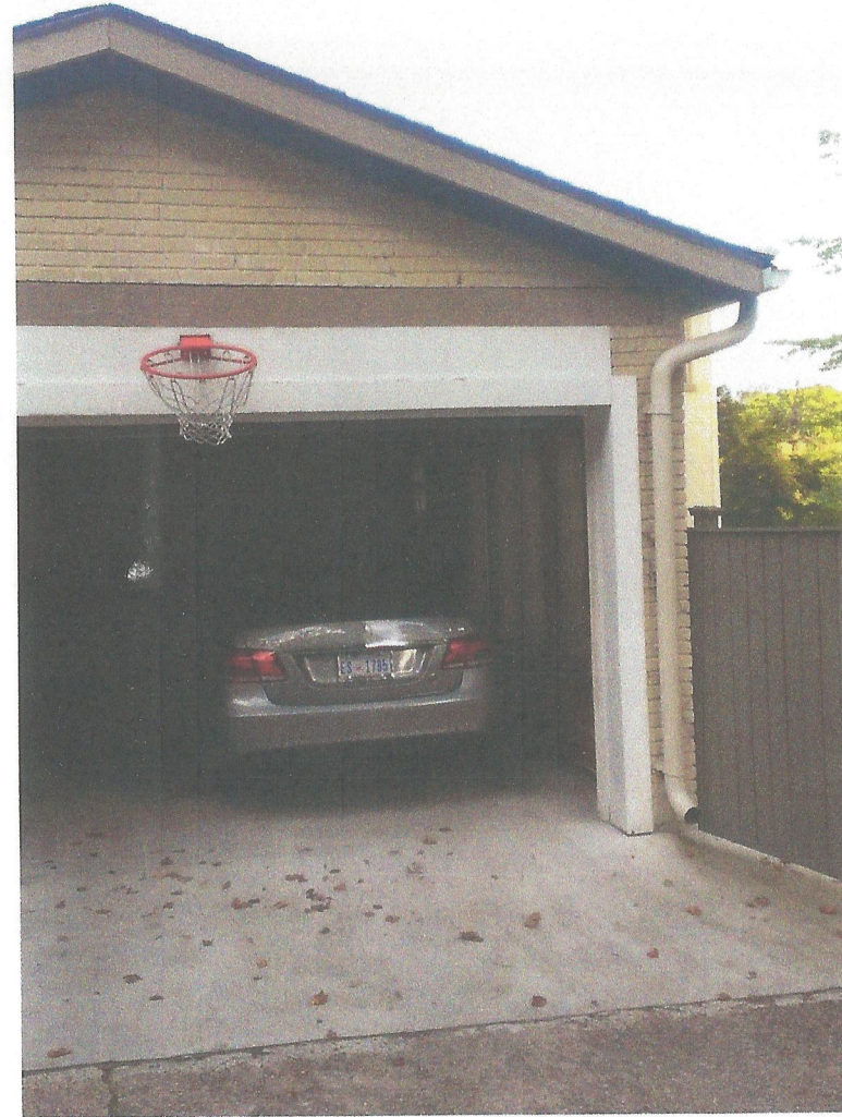
The Existing Garage; Addition Proposed on the Right of this Structure
