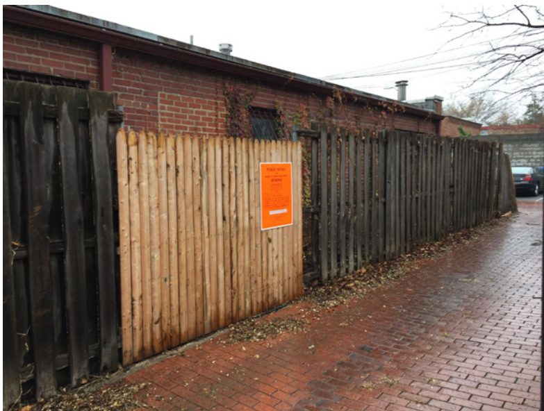
Photo #3: South facade of property, facing Browns Ct. SE (10' wide section)
