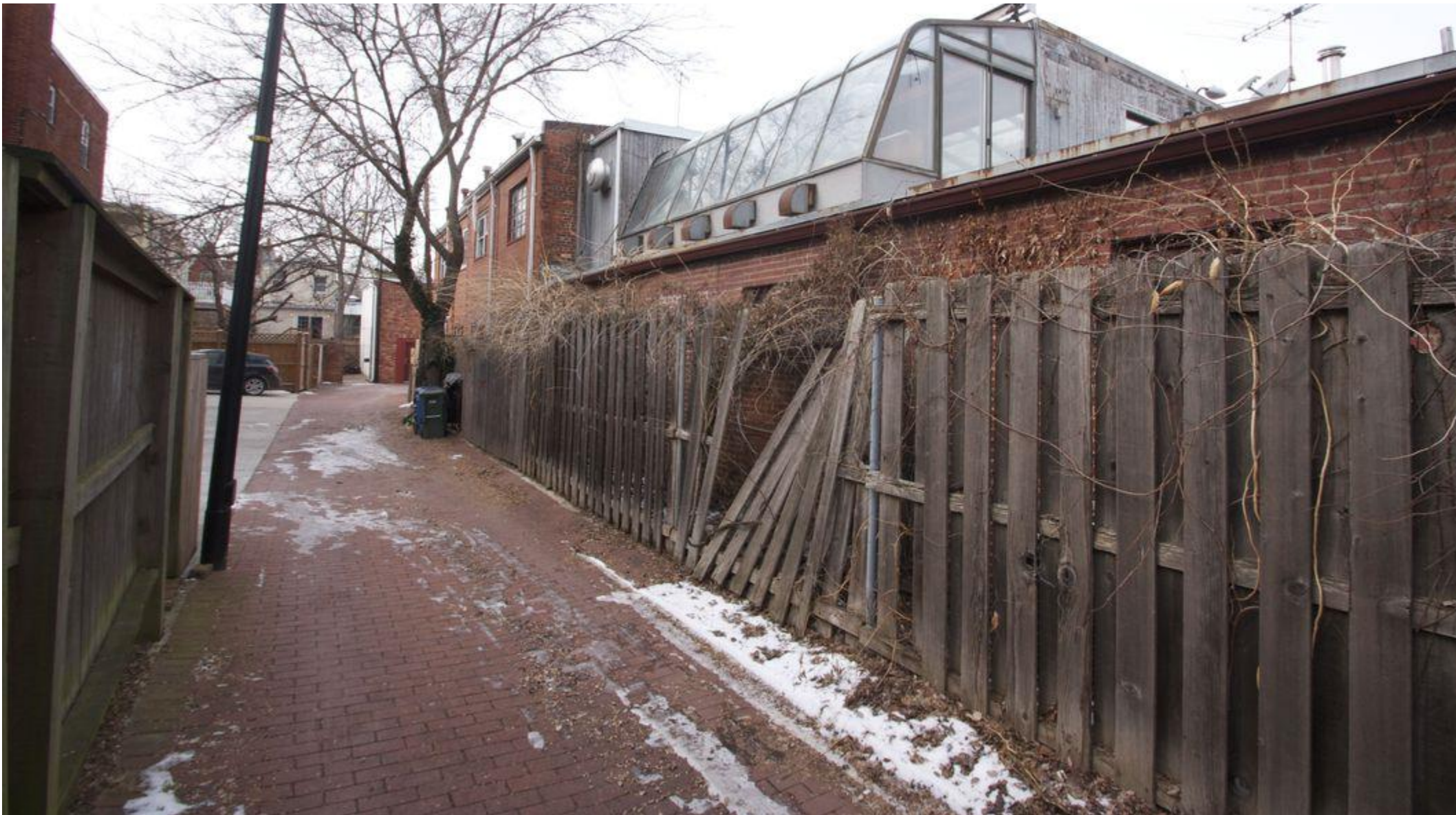
Photo 3: View along the 10' wide pedestrian alley at the south side of the site. The wood fence at right sits on the south property line. The greenhouse portion of the existing second story addition is visible.
