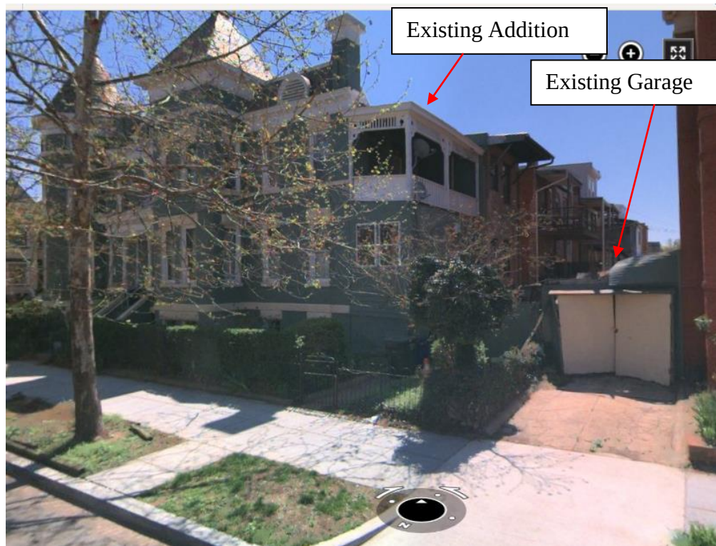
House and Garage Fronting on S Street, NW
