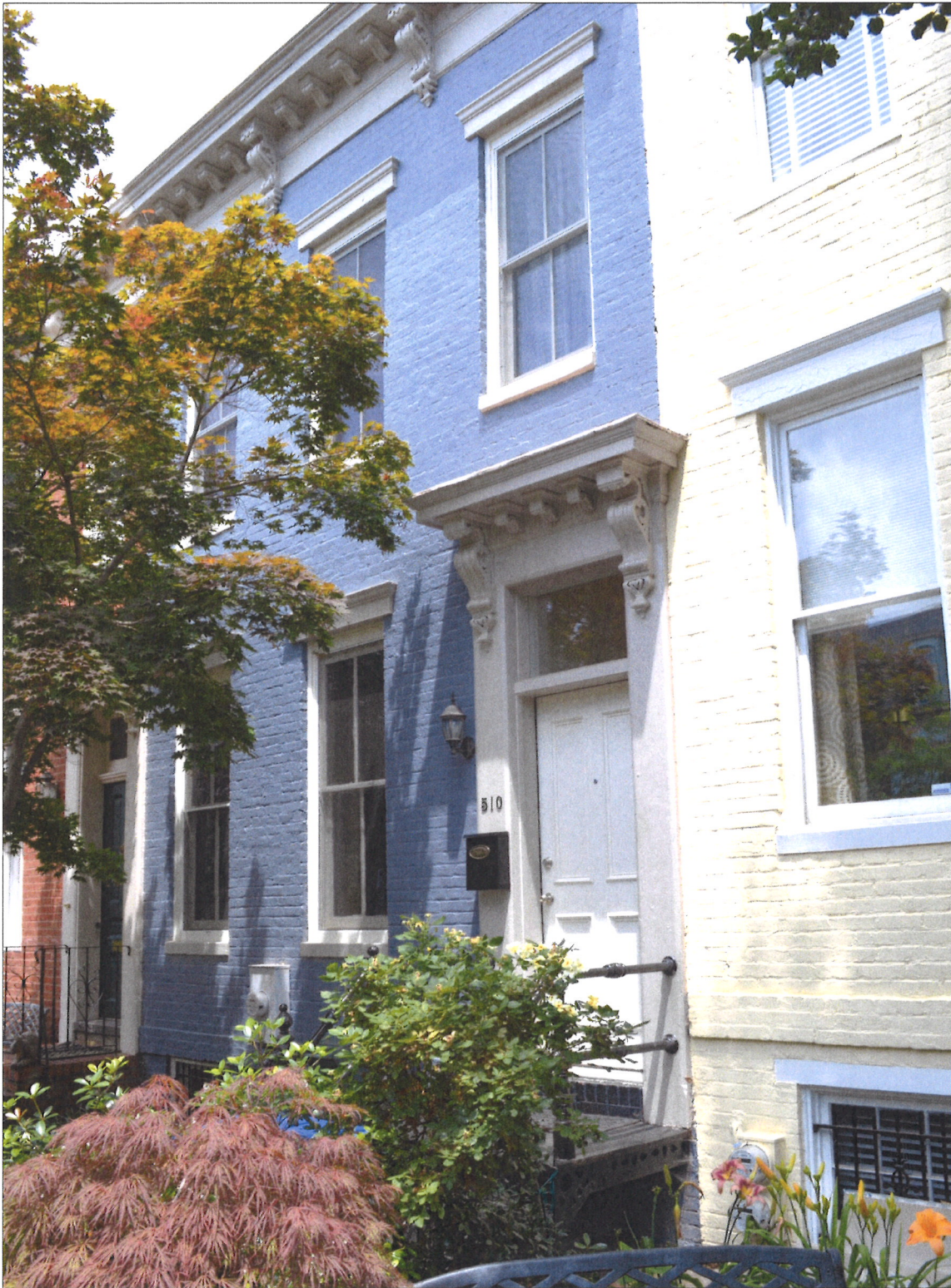
FRONT OF PROPERTY FROM INDEPENDENCE AVENUE SE
