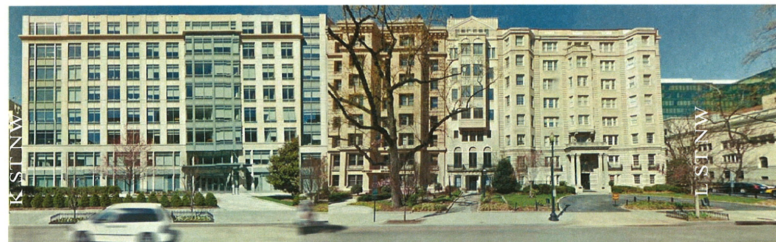
1. EXISTING CONDITION-VIEW FACING WEST ON 16TH STREET
