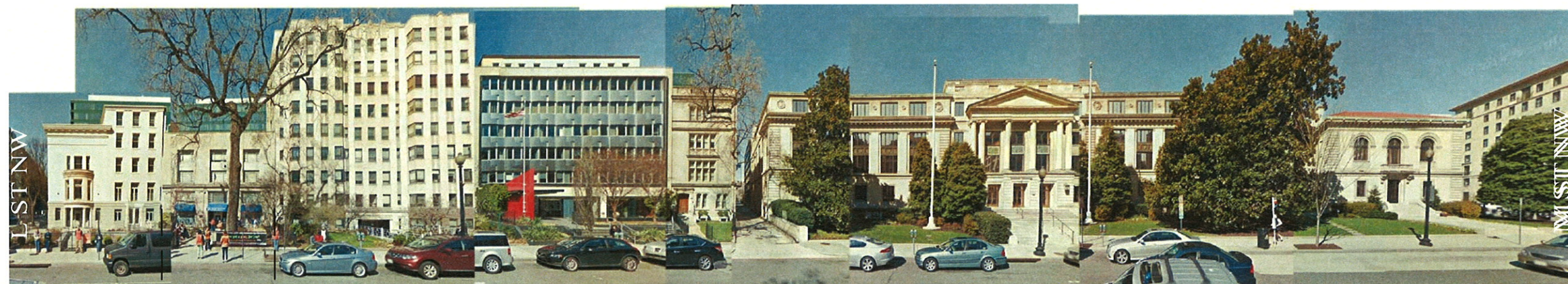
2A. EXISTING CONDITION-VIEW FACING WEST ON 16TH STREET
