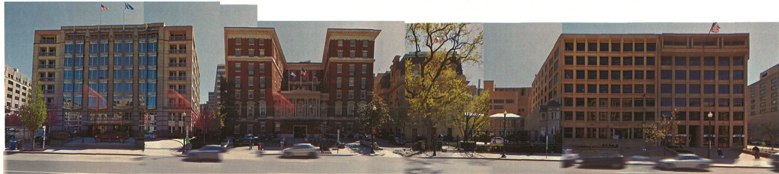
3. EXISTING CONDITION- VIEW FACING EAST ON 16TH STREET
