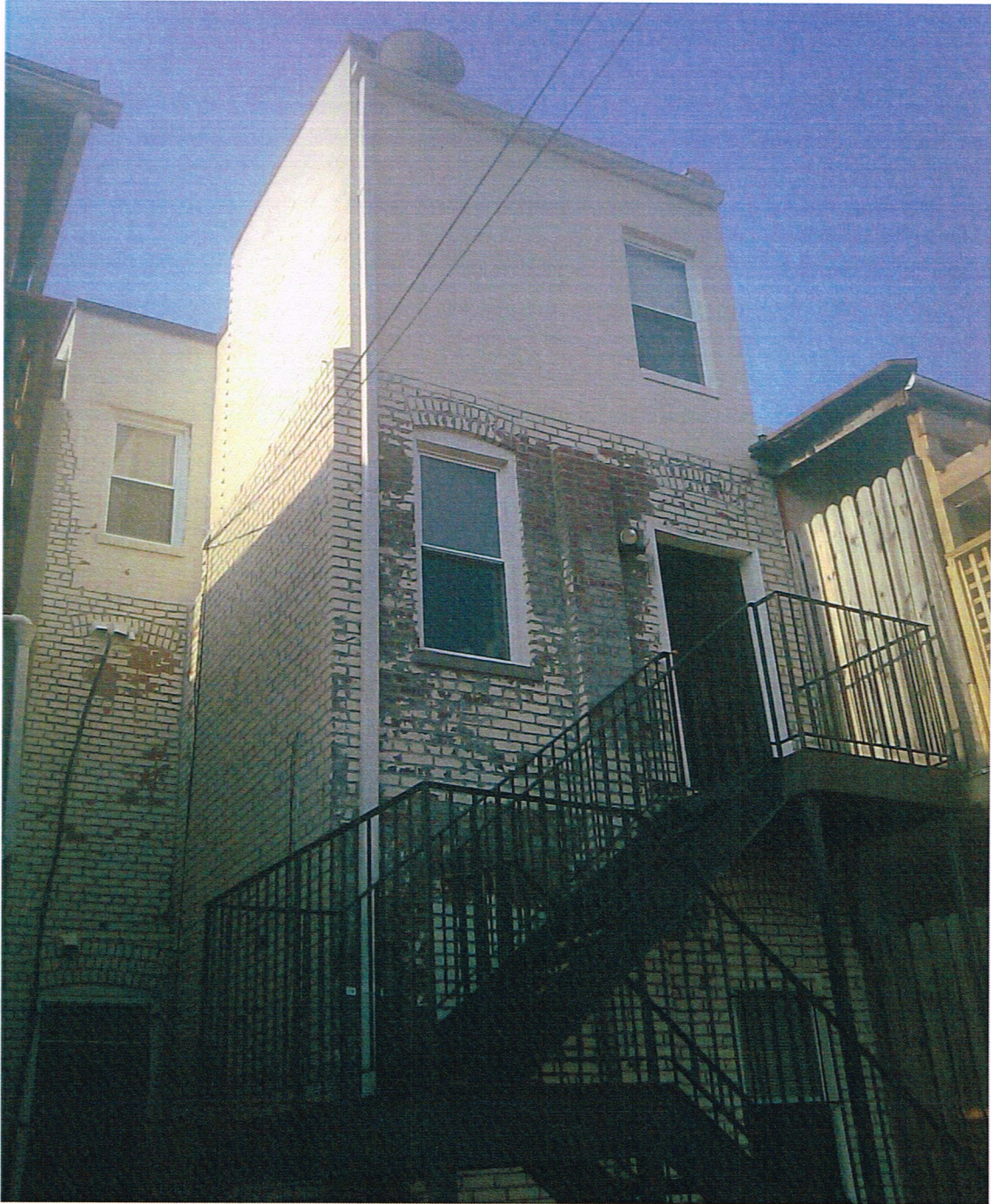
Rear of House, showing existing stoop/stair serving upper and lower doorways of house
