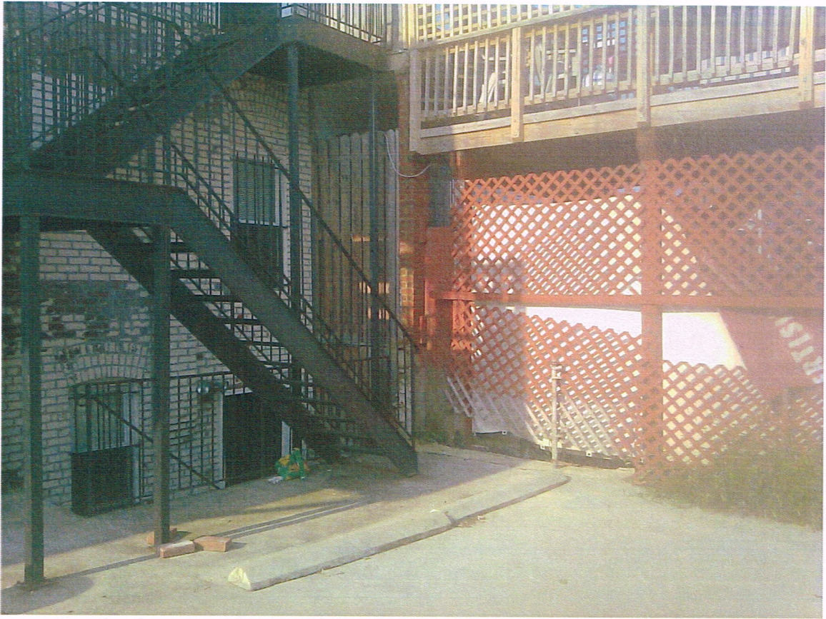
Rear of subject house, with view of existing concrete pad where occupants currently park their cars
