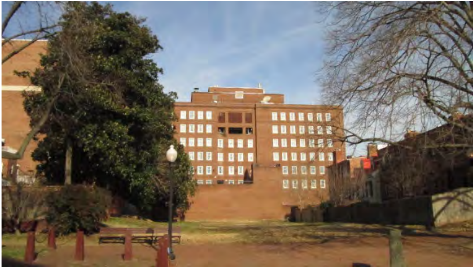
6. CANAL TOW PATH LOOKING NORTH
