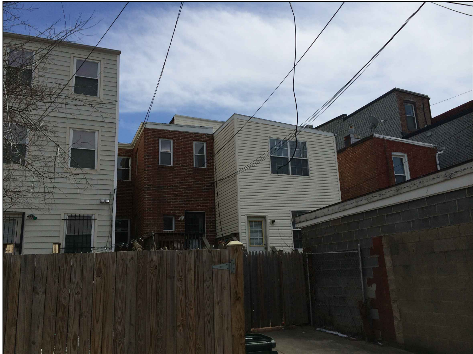
2 VIEW FROM ALLEY, LOOKING SOUTH C-6 SCALE: NTS
