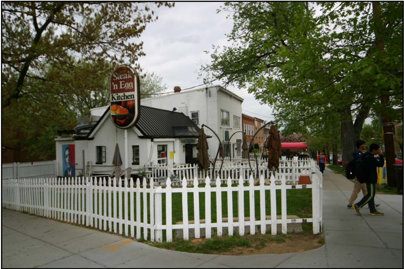
CORNER VIEW- CHESAPEAKE ST. & WISCONSIN AVE.
