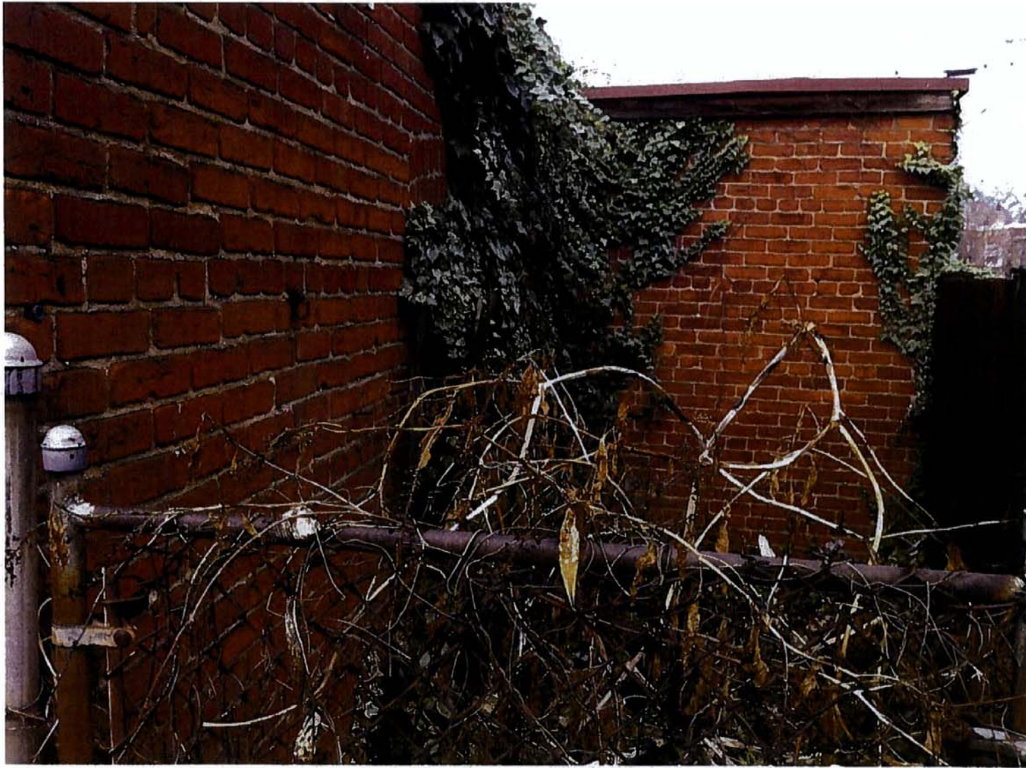
SE corner of building
