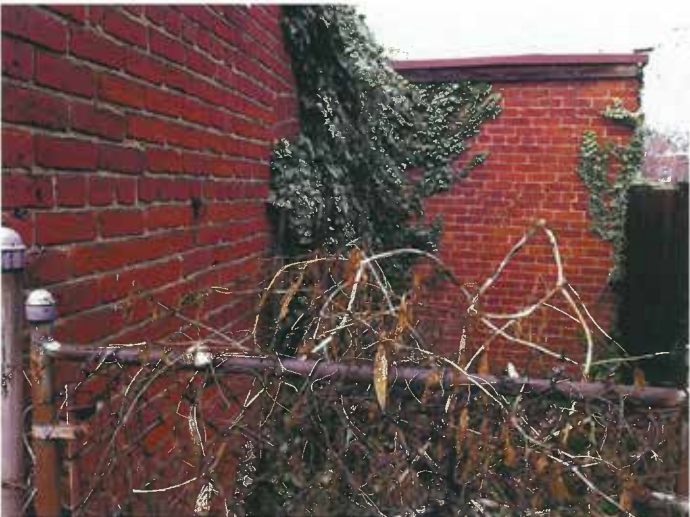
SE corner of building
