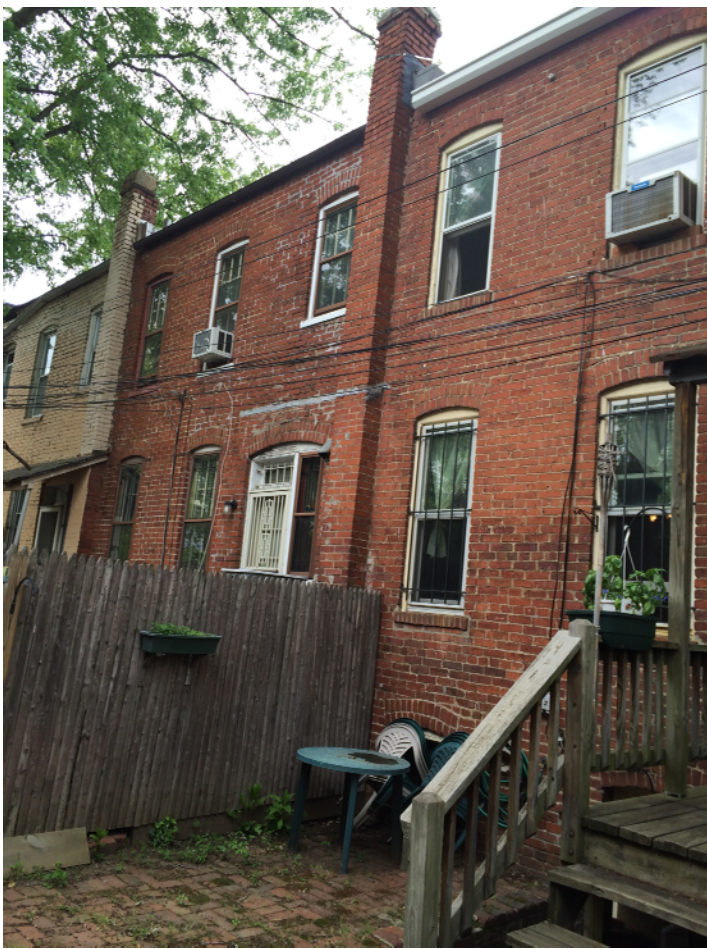
View towards the west
