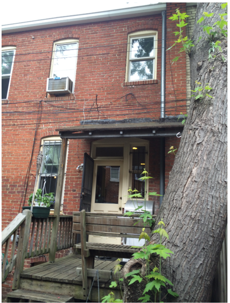
Rear of property, view from rear yard
