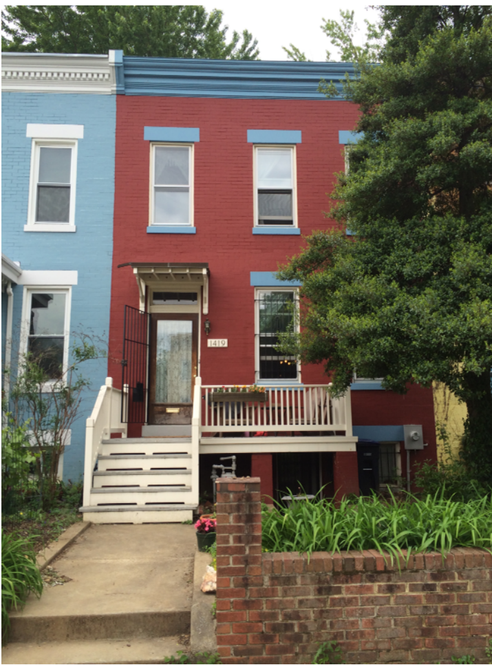
Front of property, view from F Street NE
