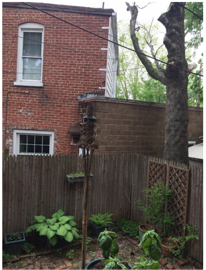
View towards the south
