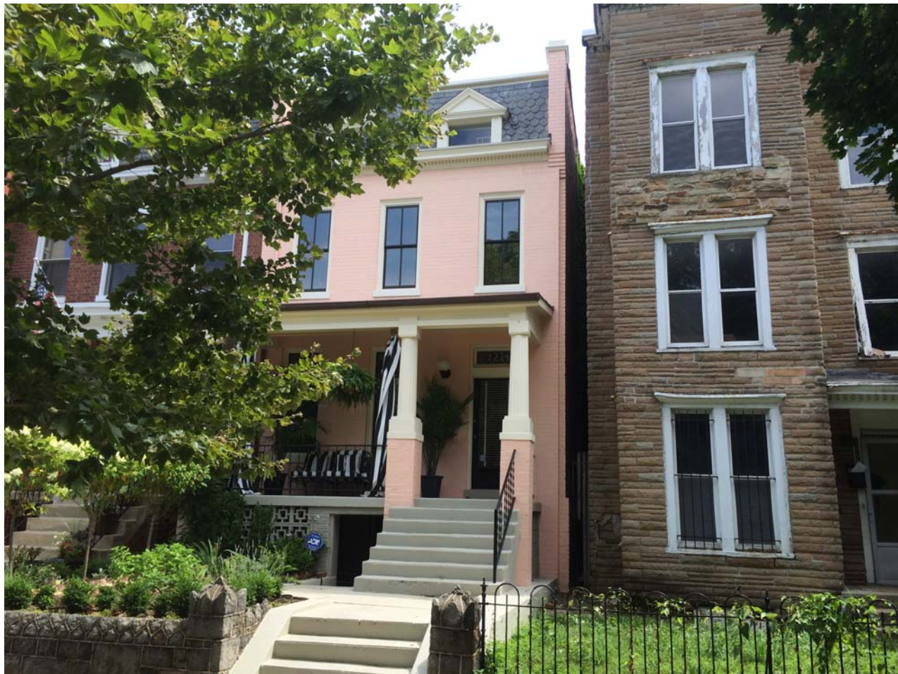
Front of house, view from F Street NE
