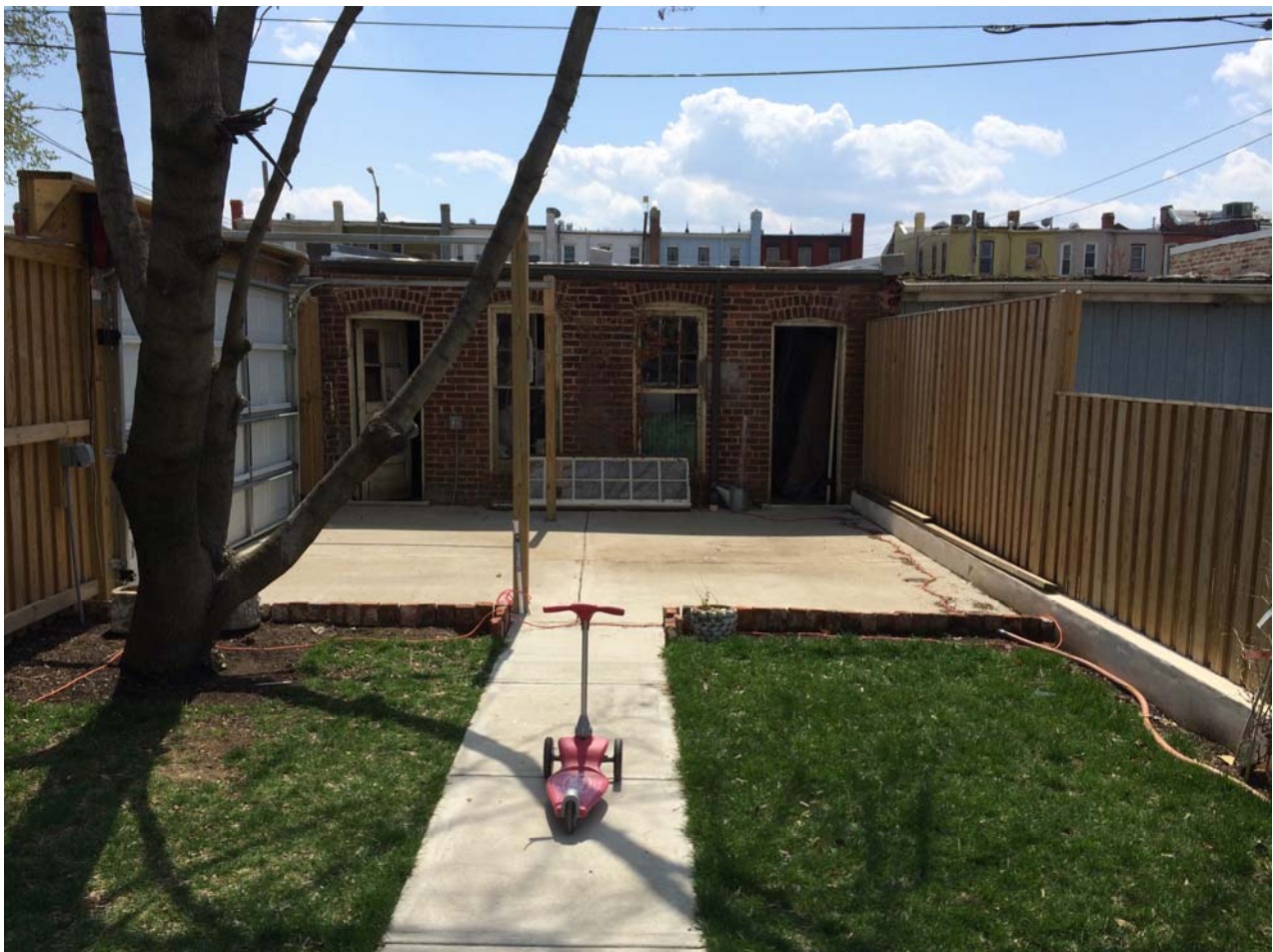
View of existing garage from grade at yard
