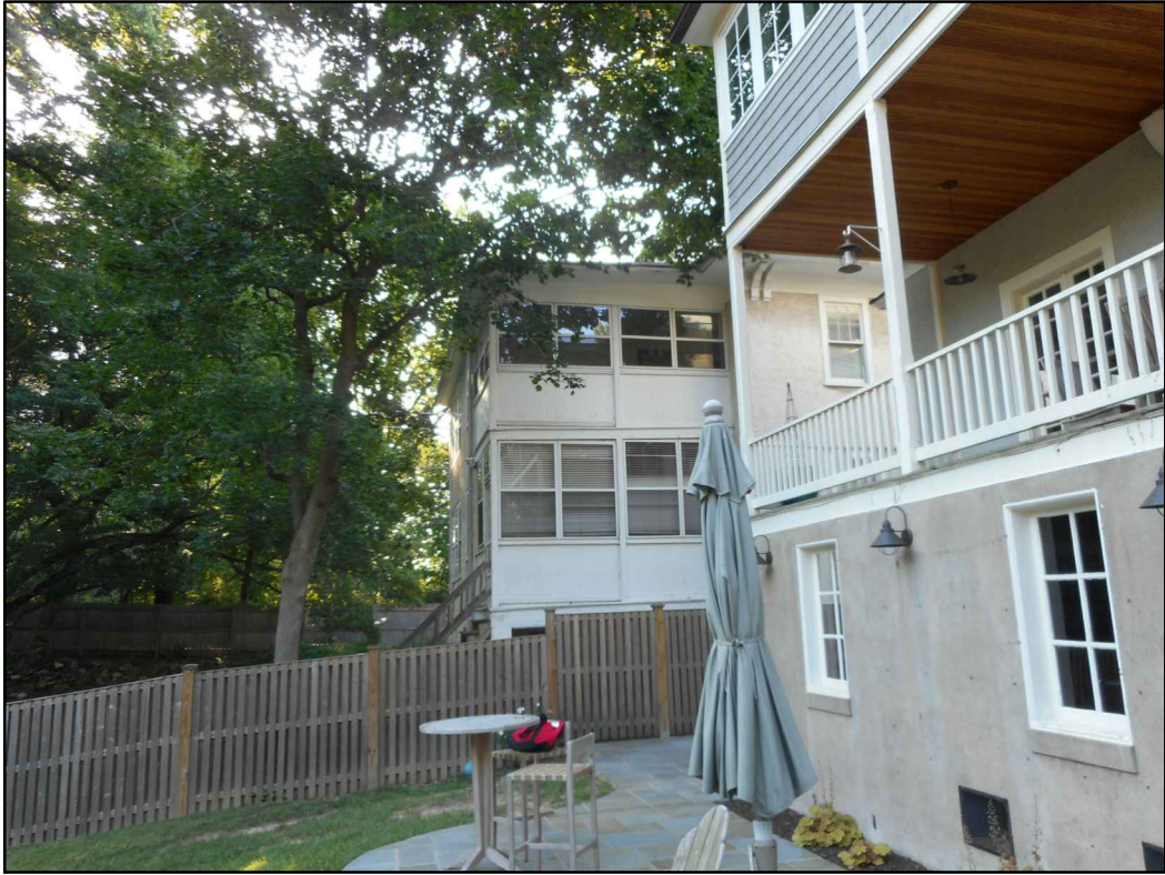
VIEW FROM EAST PROPERTY LINE (ADJACENT TO PUBLIC PLAYGROUND) AREA OF ADDITION NOT VISIBLE IN THIS IMAGE
