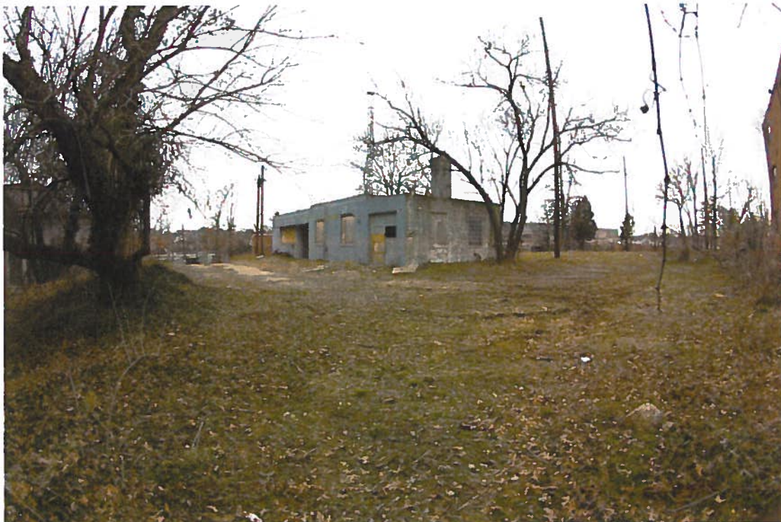
STANDING AT THE SOUTHEAST PORTION OF THE SITE LOOKING NORTH/ NORTHWEST (Opposite corner from existing drive/ curb cut).
