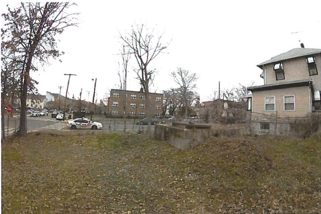
STANDING ON THE NARROW PORTION OF THE SITE, CLOSE TO TRENTON STREET, Showing the intersection of Trenton Street SE and 4th Street SE, residential properties on the east and across Trenton street.
