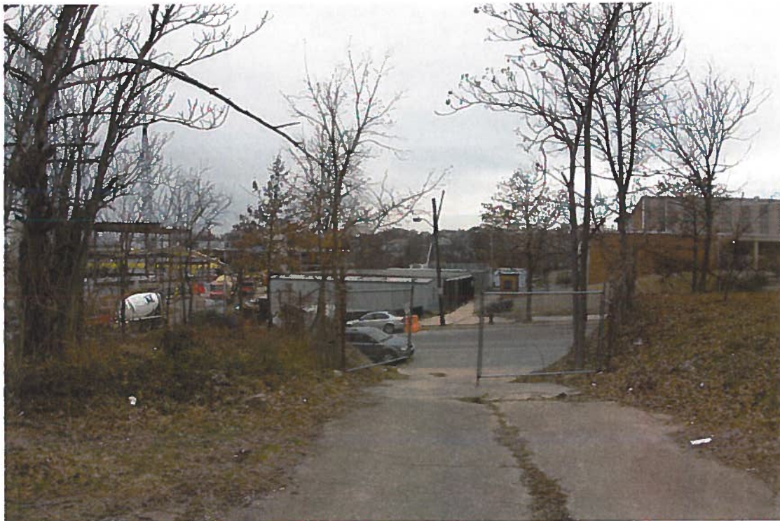
ON TOP OF EXISTING DRIVE LOOKING WEST, Showing 4th Street; on-going construction of the new Ballou Senior High School on the left, and existing Ballou Senior High School on the right.
