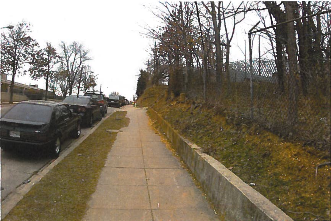
ON 4TH STREET SE, Southwest corner of the property looking North (along 4th street towards Trenton Street). Showing chain link fence, sidewalk, 18" concrete retaining wall and retained earth.
