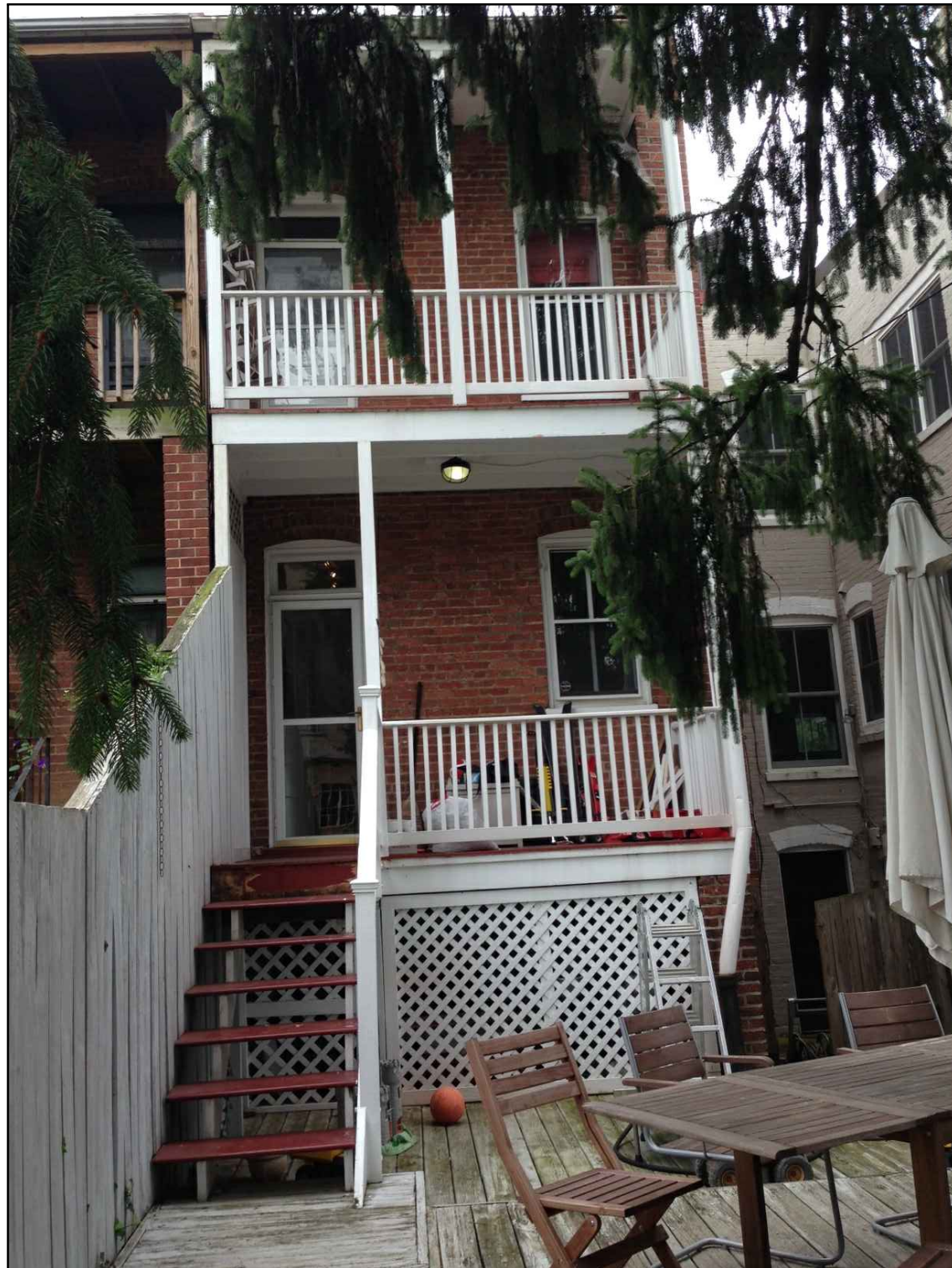
2 REAR OF HOUSE, VIEW FROM YARD C-4 SCALE: NTS
