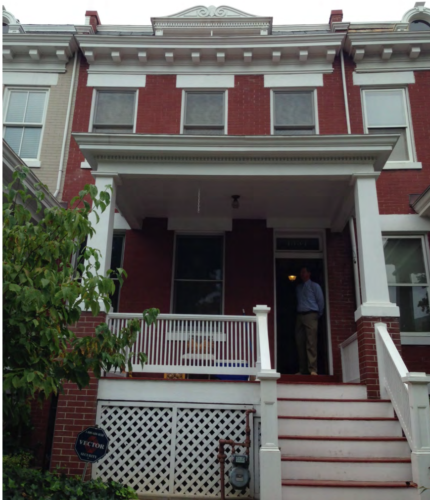
FRONT OF HOUSE, VIEW FROM A STREET SE
