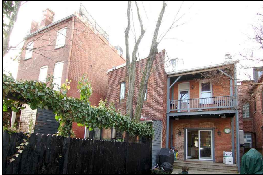
3 View from Backyard looking Southeast N.T.S.
