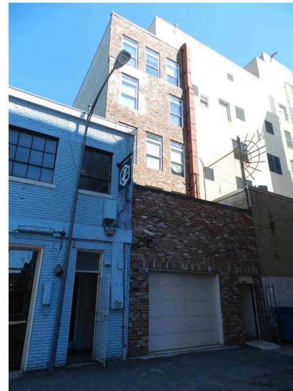
EXISTING VIEW OF 1712 14TH STREET NW REPRESENTING PRECEDENT FOR MASSING AND SCALE ALONG ALLEY
