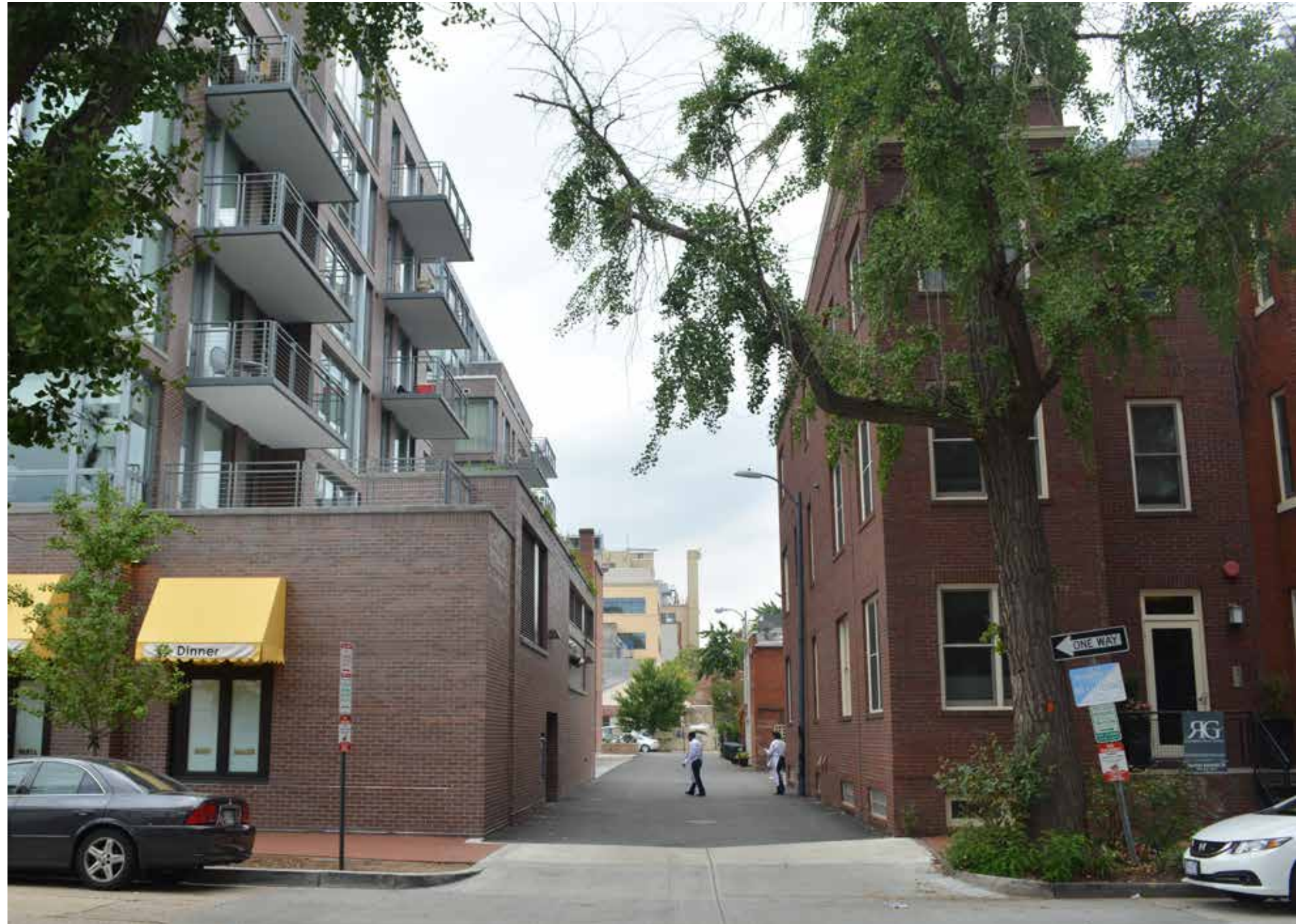
EXISTING VIEW OF ALLEY BEHIND 1810 14TH STREET NW
