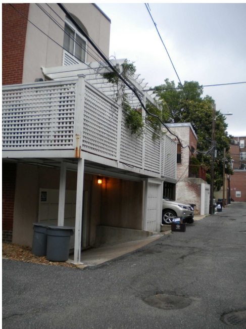
D. ALLEY - LOOKING EAST
