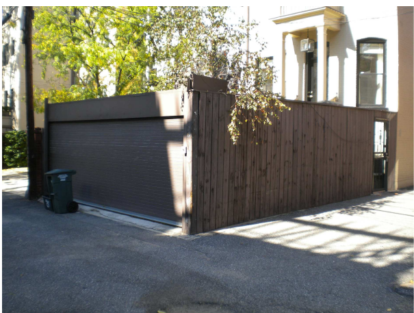
I. ALLEY - EXISTING REAR ENCLOSURE
