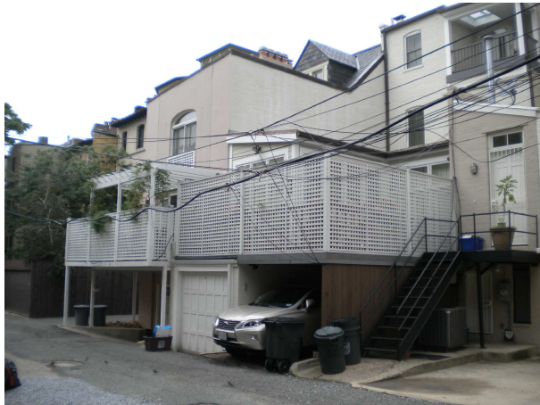
A. ALLEY - LOOKING WEST
