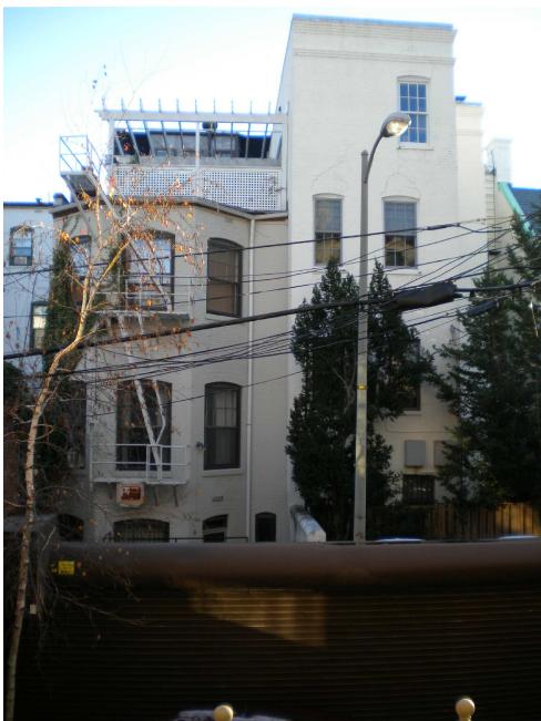
E. ALLEY - LOOKING SOUTH OF RESIDENCE
