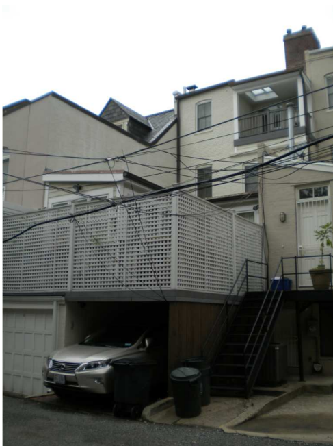
B. ALLEY - NORTH WEST
