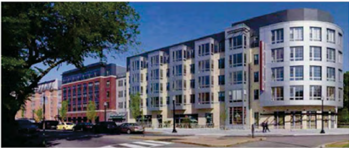
JENKINS ROW (1391 PENNSYLVANIA AVENUE, SE) 4-STORY CONDOMINIUM COMMUNITY WITH 247 UNITS. COMPLETED IN 2007, THE PROPERTY INCLUDES ROOF DECKS, A FITNESS CENTER, A GROUND-FLOOR HARRIS TEETER, AND MUCH MORE.
