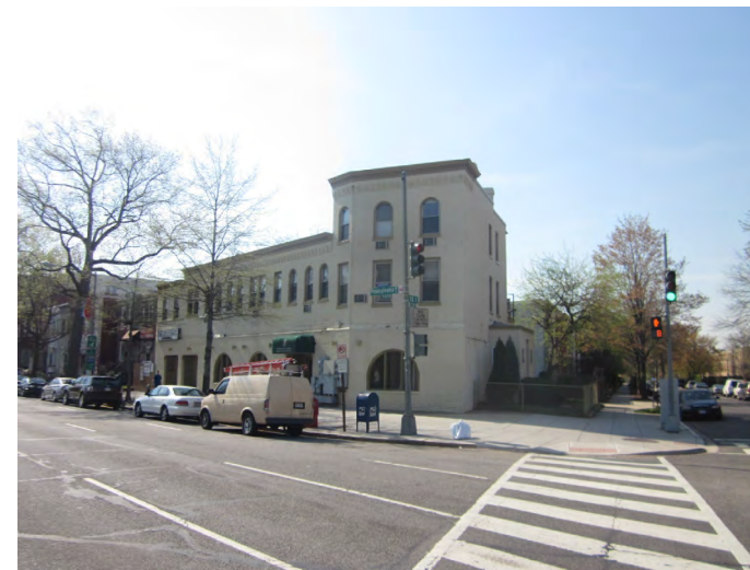
PENNSYLVANIA AVENUE LOOKING SOUTH 3
