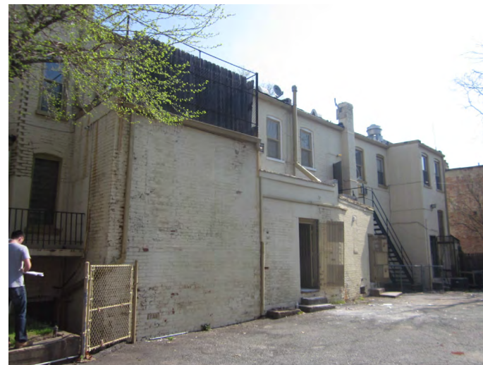
13TH STREET LOOKING NORTHEAST 6
