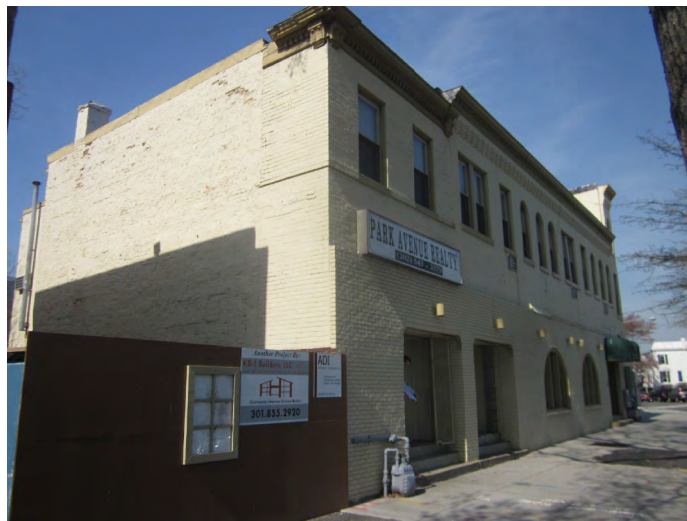
PENNSYLVANIA AVENUE LOOKING WEST 1
