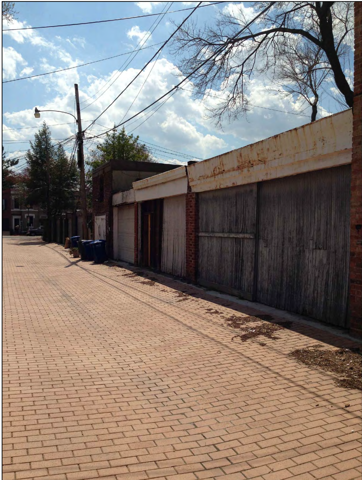
2 VIEW FROM ALLEY, LOOKING SOUTH C-6 SCALE: NTS
