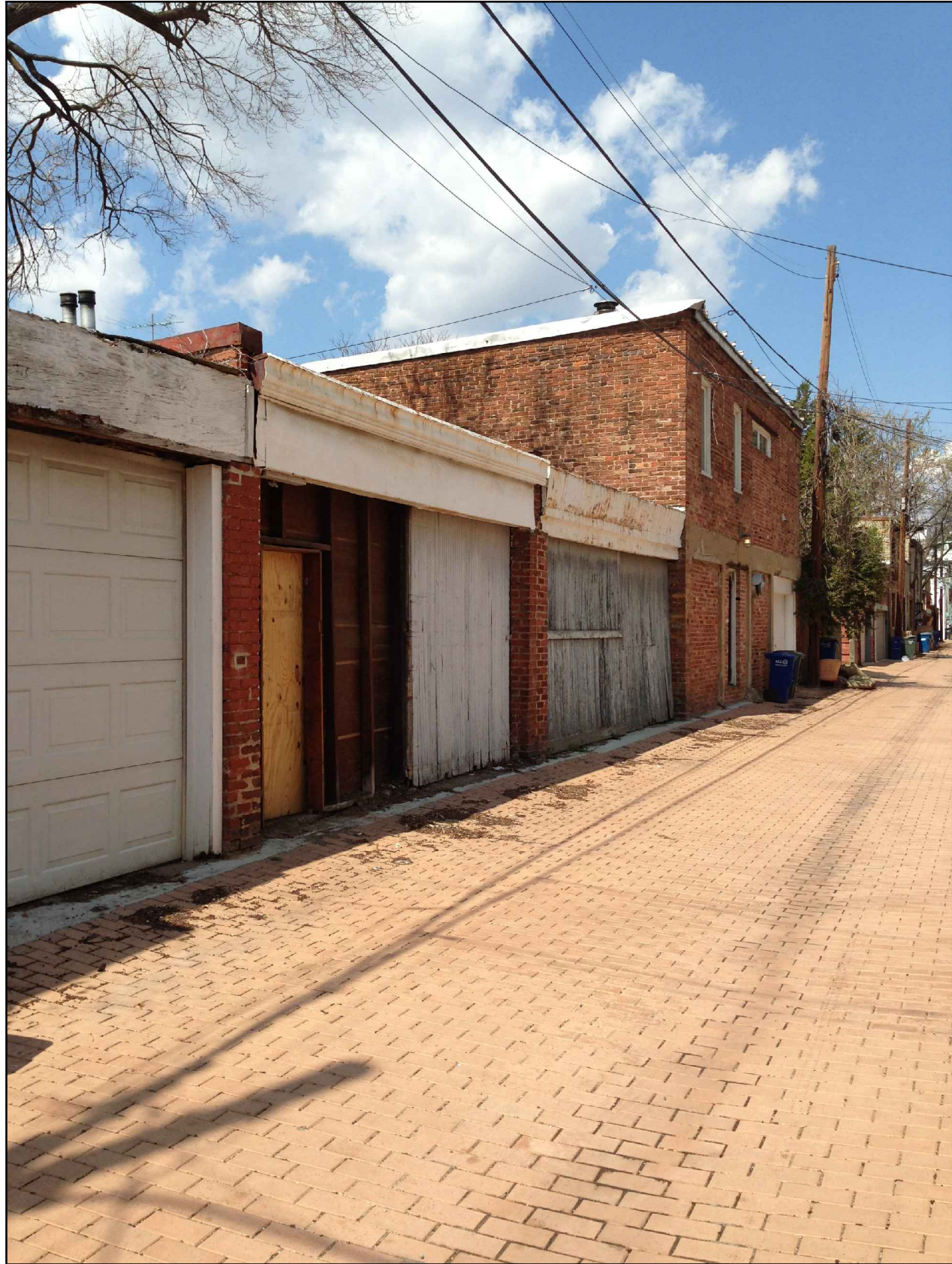
1 VIEW FROM ALLEY, LOOKING NORTH C-6 SCALE: NTS
