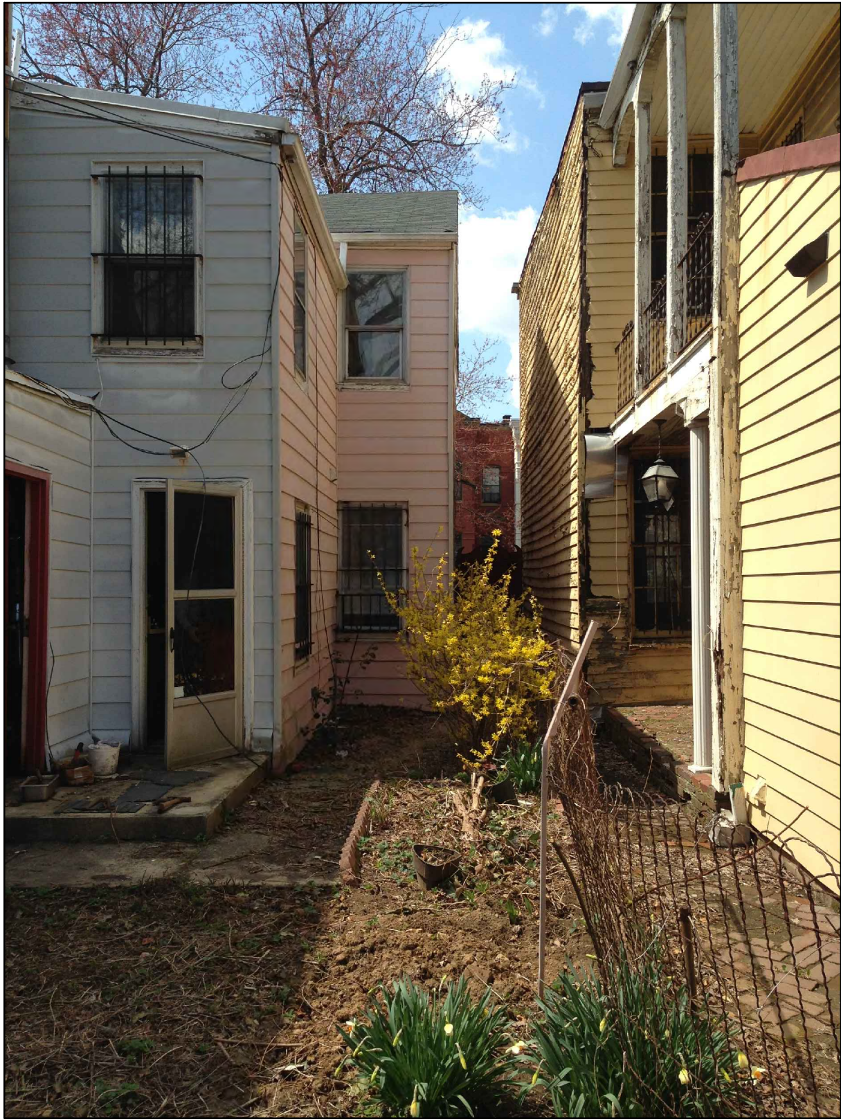
1 VIEW THROUGH SIDE YARD, FROM REAR YARD C-5 SCALE: NTS
