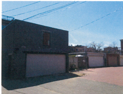
View 2 of site from alley
