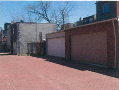
View 1 of site from alley
