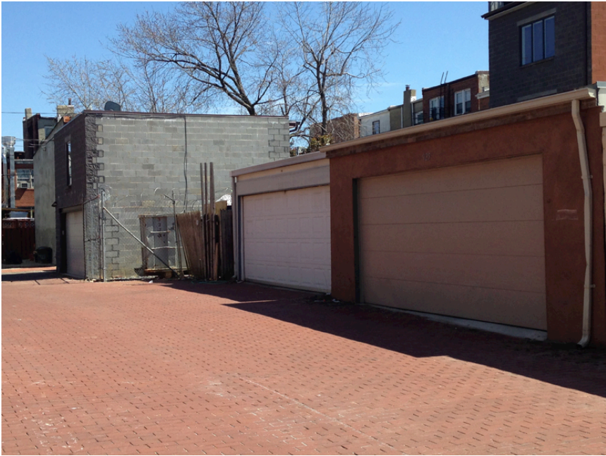
View 1 of site from alley
