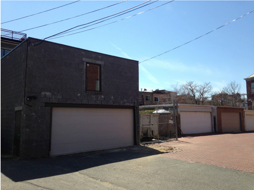
View 2 of site from alley
