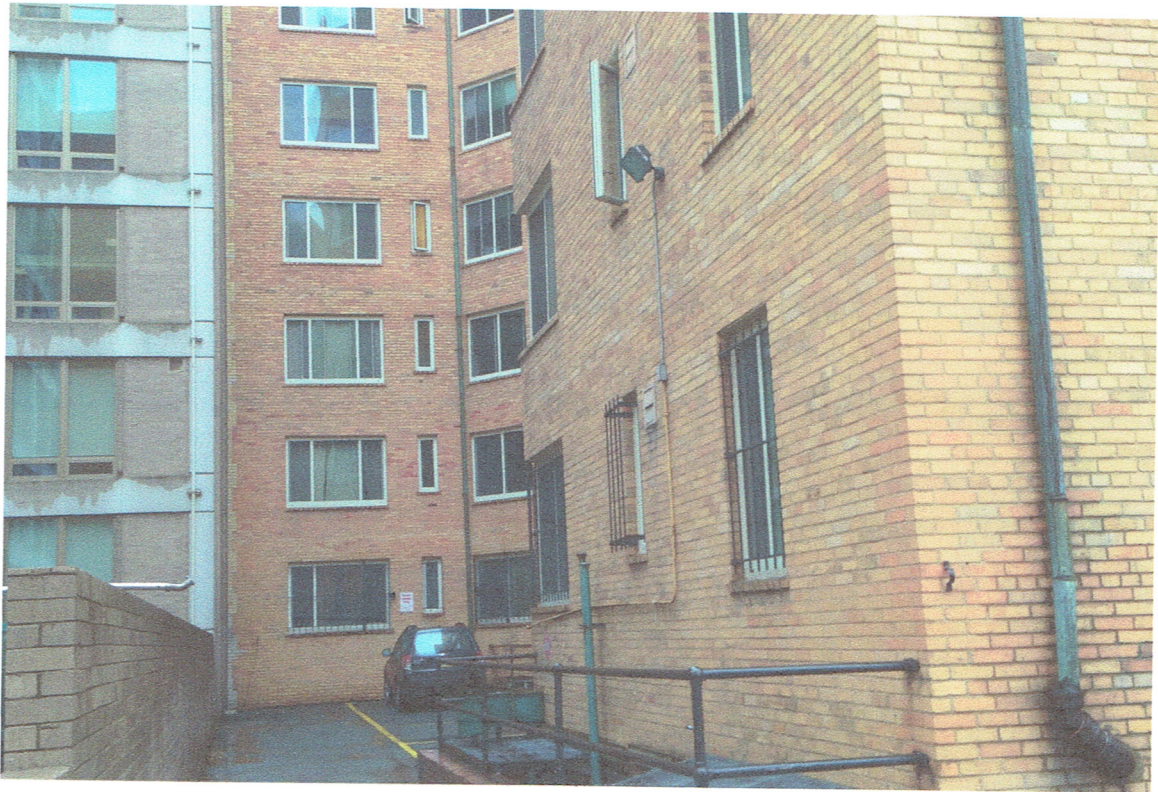
PHOTO 2 VIEW FROM REAR ALONG EAST SIDE
