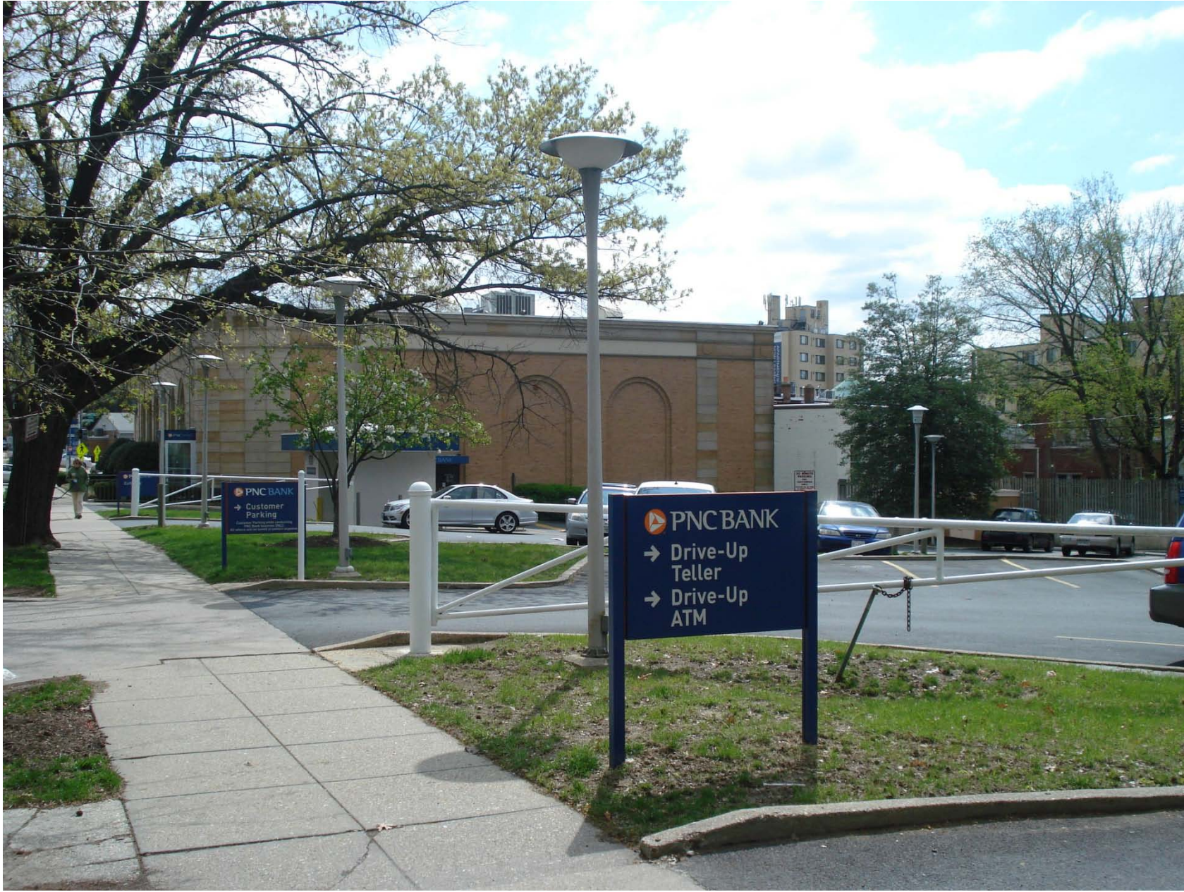
Photograph from Morrison Street Facing Southeast
