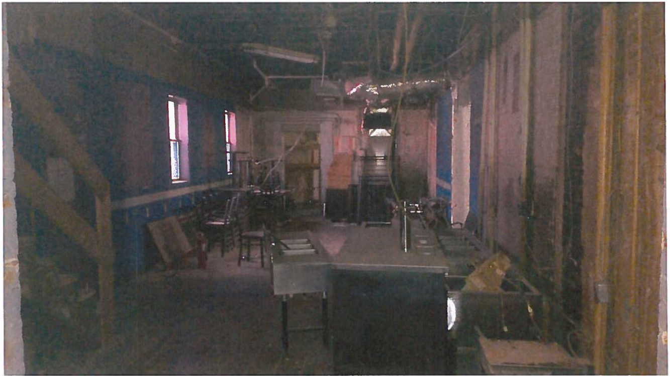
Interior View of the Subject Building
