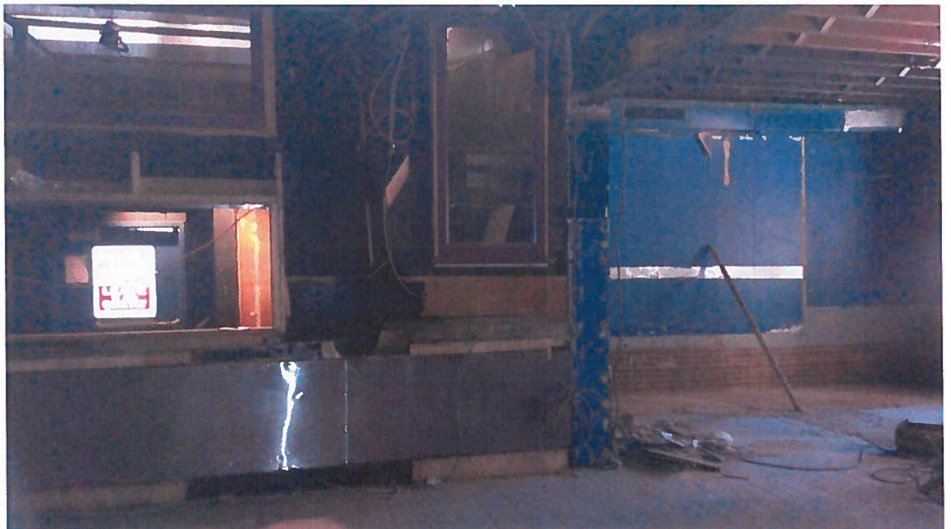
Interior View of the Subject Building
