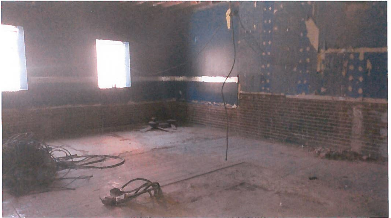
Interior View of the Subject Building
