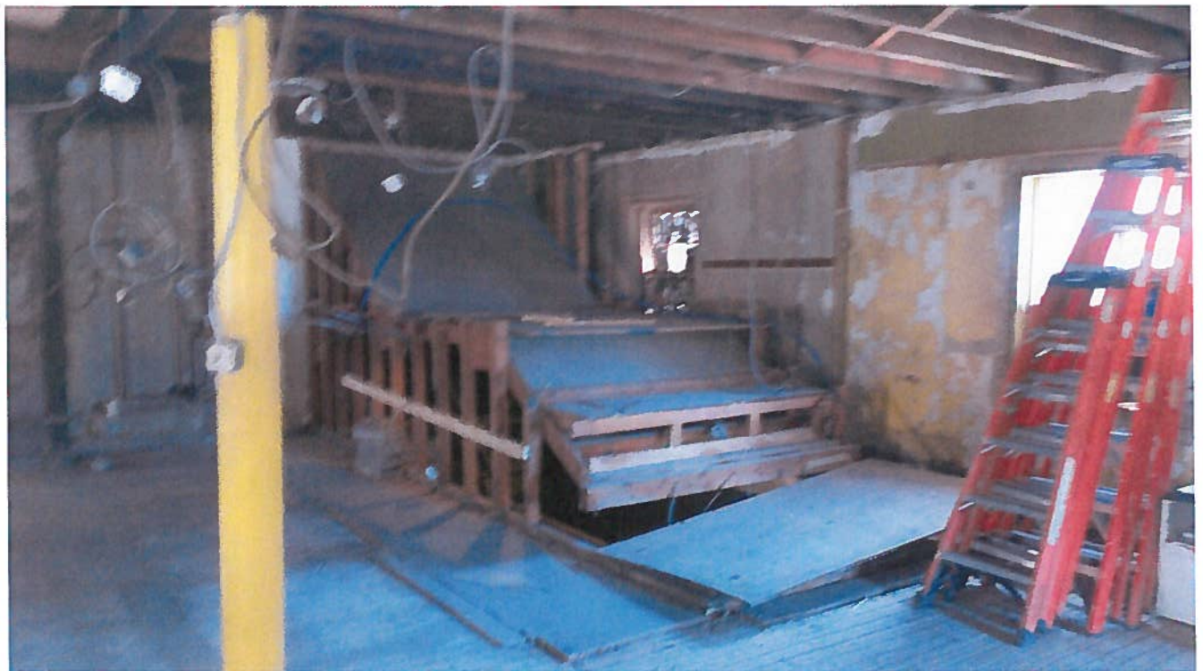
Interior View of the Subject Building
