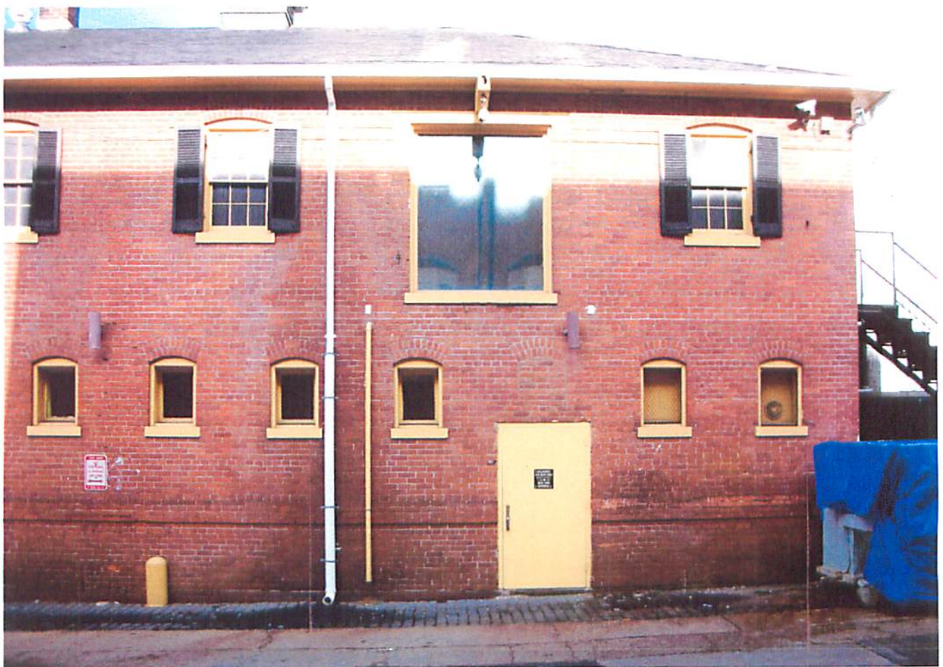
HAY DOOR & BLOCKED STALL WINDOW
