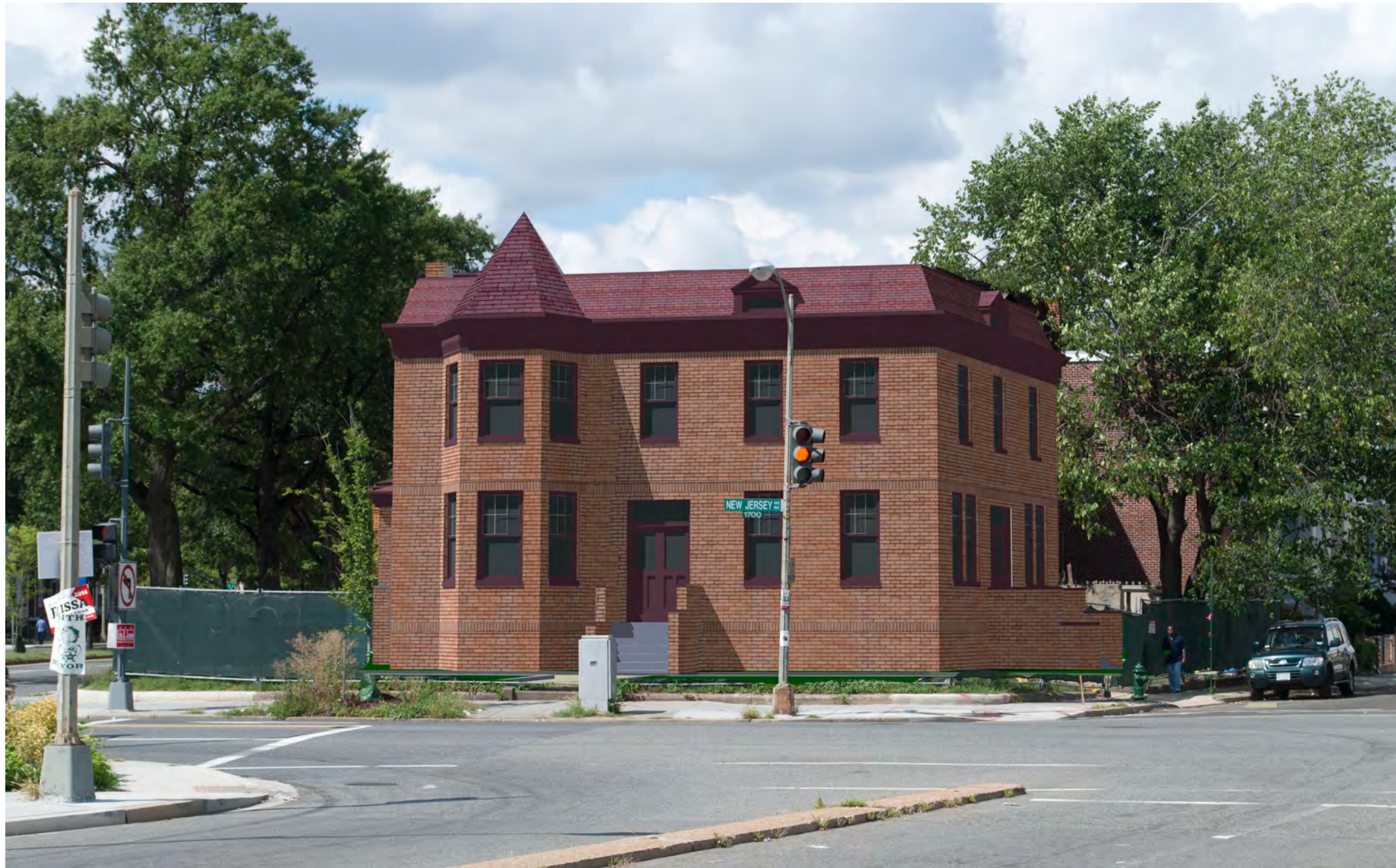
EXISTING CONDITIONS - LOOKING WEST
