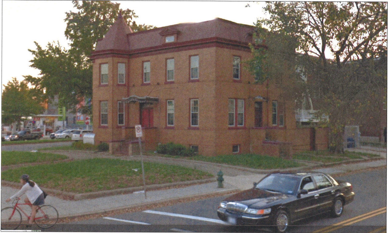
FACING SOUTHWEST FROM NEW JERSEY AVE & S STREET NW
