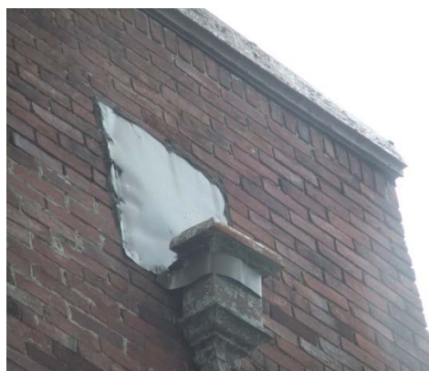
Photo 27: Disconnected drain scupper at northeast corner of the building.
