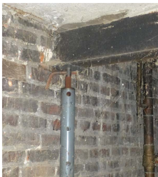
Photo 8: Steel post shore positioned beneath a steel beam presumably to provide support for a compromised bearing condition at the exterior masonry wall
