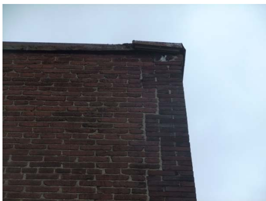
Photo 24: Toothed wall construction at southeast corner of the building, tying the south and east facades together.
