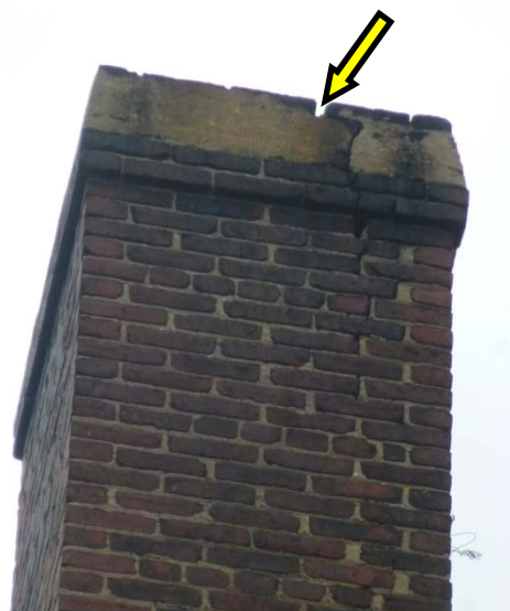
Photo 30: Deterioration of parging and cracks through the chimney cap.
