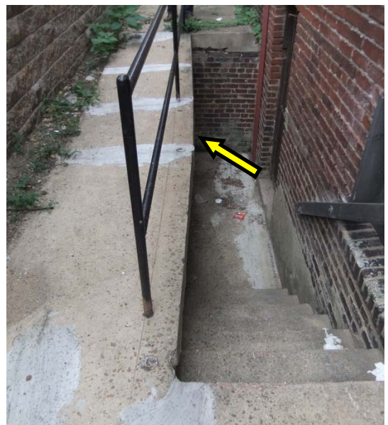
Photo 22: Exterior stairwell at west façade with horizontal bow noticeable in brick retaining wall and exterior slab on grade.
