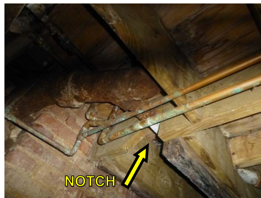
Photo 11: Floor joist notched for passage of drain line.
