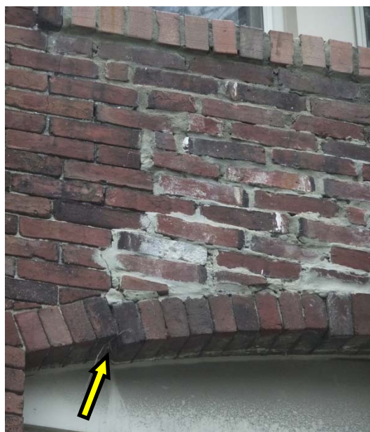
Photo 26: Displaced brick arch with previous repair at the east façade.
