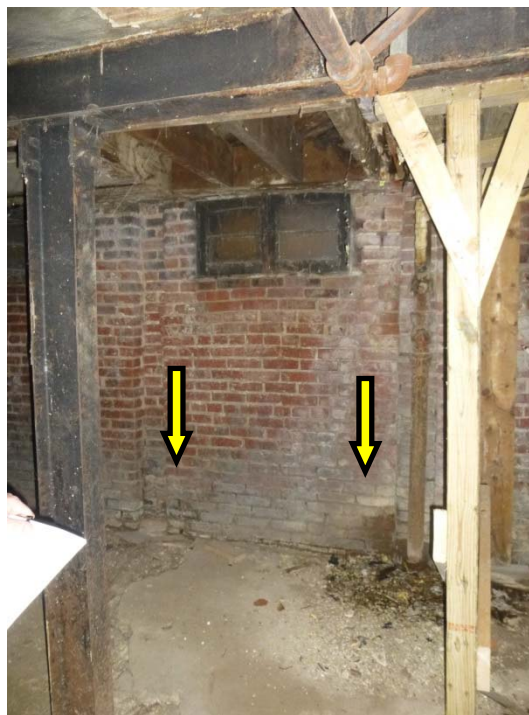
Photo 5: Settlement of the foundation wall at either side of the basement window which faces the entrance walkway. Note the temporary wood shoring at the right edge.
