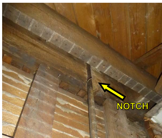
Photo 16: Full depth notch in outer ply of built-up wood beam above the north wall of living room in Unit D to the south of the main stair on the first floor.
