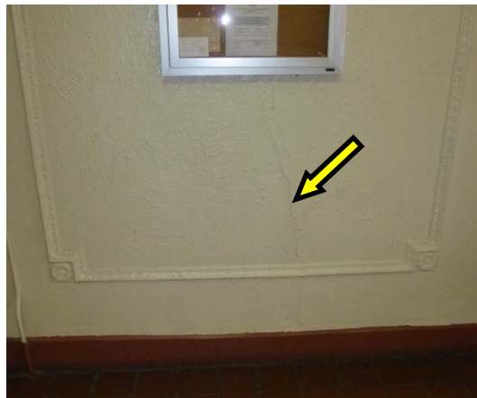
Photo 14: Plaster repair of crack on north wall of lobby.
