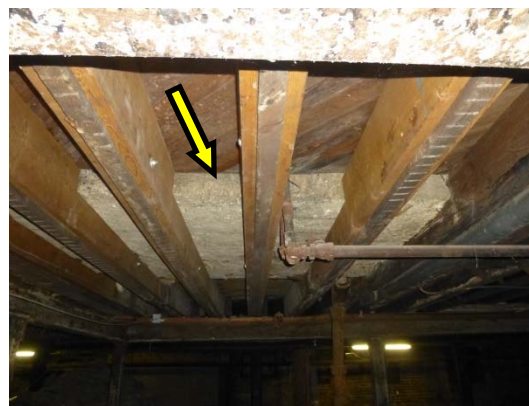
Photo 12: Original fire damaged joists with wood sister at either face. Note that the sisters have been notched to incorporate the additional cementitious material.
