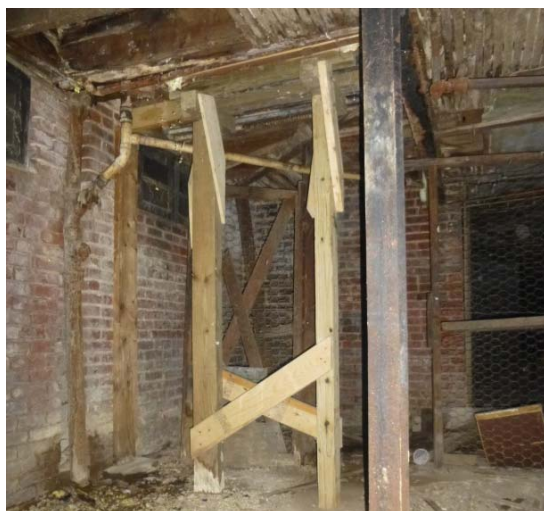
Photo 9: Temporary shoring structure for support of wood framing above.
