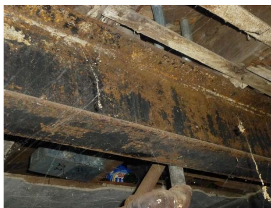
Photo 7: Corrosion of steel beam in north east quadrant of building.
