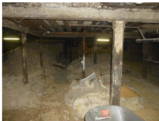
Photo 2: View of northern half of basement level showing piles of debris from slab on grade removal. Note the steel beam and column lines.
