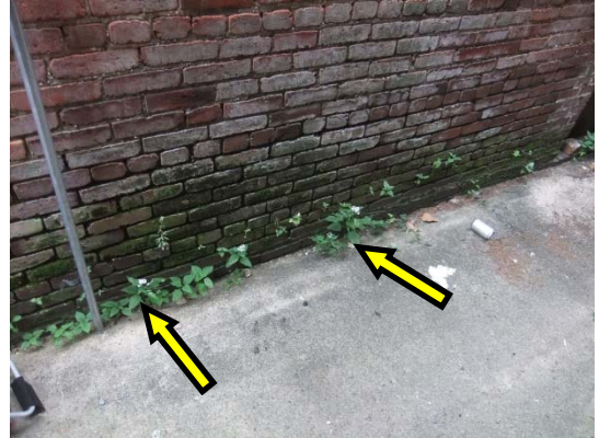
Photo 21: Vegetation growth along the base of the exterior masonry at the west façade.
