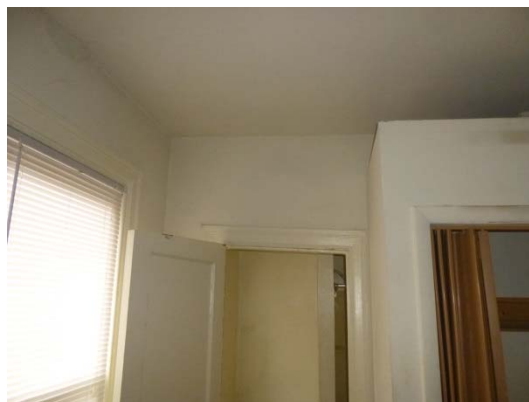
Photo 18: Racking of bathroom doorframe in Unit F on the second floor.
