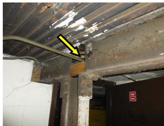
Photo 13: Atypical beam framing at top of steel column; the steel beam is not continuous over top of the column.
