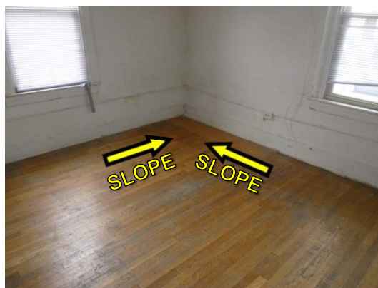
Photo 15: Floor slopes toward northeast corner of living room in Unit A at the northeast corner of the first floor.
