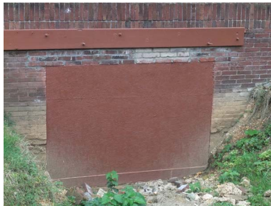
Photo 28: Opening at base of exterior foundation wall along the north façade has been covered with plywood.
