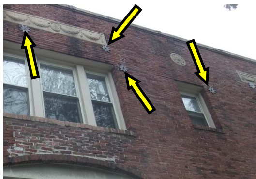
Photo 25: East façade of building showing locations of star anchors.
