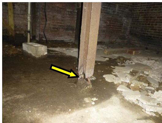
Photo 6: Steel support column in the southwest quadrant of the basement with nearly full section loss at its base.
