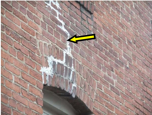
Photo 20: Brick arch at the south façade with displaced brick. Note the white caulking used in an attempt to repair the deteriorated mortar.
