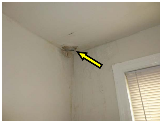
Photo 19: Water damage at ceiling of bedroom in Unit A at the southeast corner of the second floor
