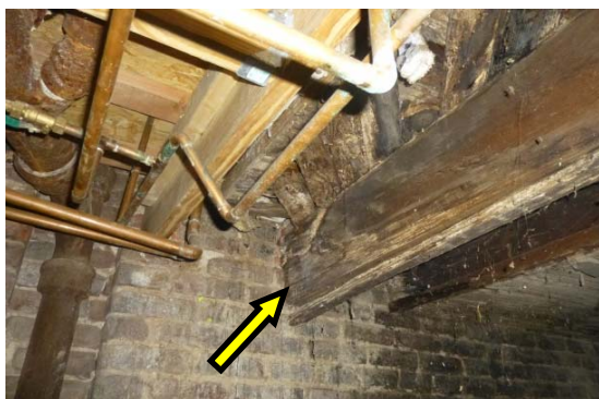
Photo 10: Wood joist with full bearing loss at west exterior masonry wall.
