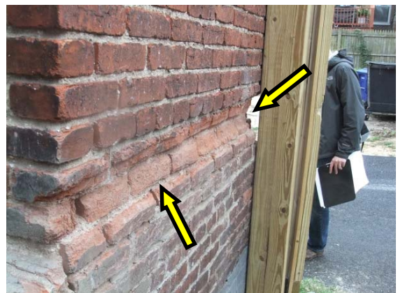
Photo 23: Brick damage at southwest corner of building
