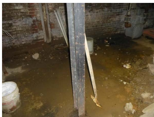
Photo 3: Ponding water visible at the slab on grade in the northwest corner of the basement.
