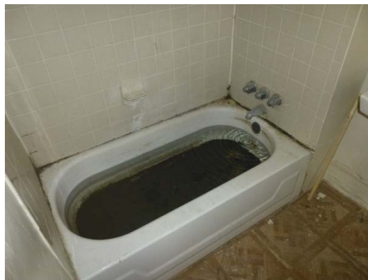
Photo 17: Bath tub in Unit D. Note that the tub does not appear to be draining.
