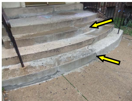
Photo 29: Cracked and spalled concrete on the exterior stairs at the entry to the building.
