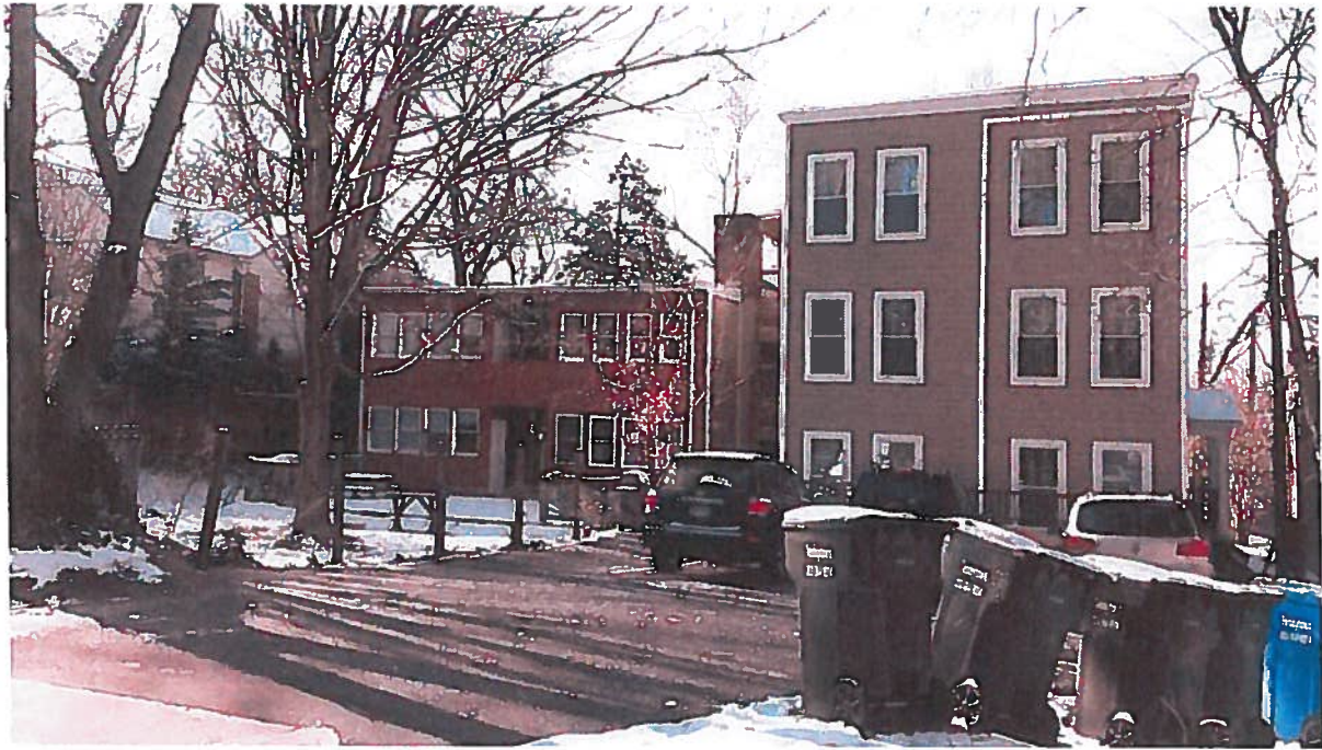
Rear of 3921 and 3925 Fulton
