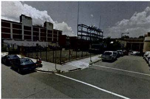
PEPCO Facility along Ontario Rd, Facing SW
