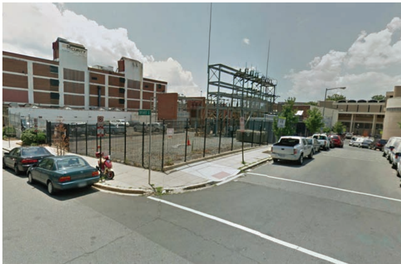
PEPCO Facility along Ontario Rd, Facing SW
