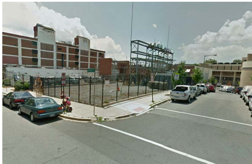
Pepco Facility Along Ontario Rd, Facing SW
