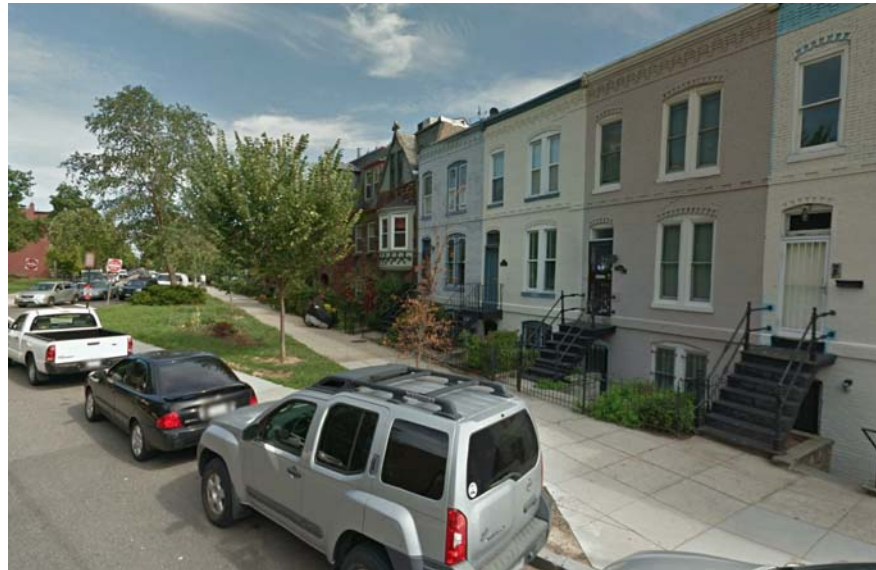
Townhomes Along Florida Ave & V Street , Facing SE
